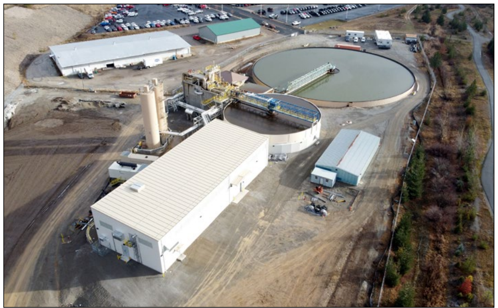
The upgraded Bunker Hill Central Treatment Plant includes the filter and polymer feed building (foreground), high density sludge thickener tank (center), and lime/polymer reactor structure (to the left of Sludge Thickener).
