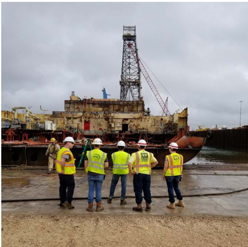
Team site visit in February to shipbreaking operations in Brownsville (l to r – APTIM Program Manager Steve Moran, International Shipbreaking Limited President Chris Green, APTIM Project Manager Sudhakar Matlapudi; Radiological Health Physicist Hans Honerlah, U.S. Army Corps of Engineers, Baltimore District, Project Manager Brenda Barber, U.S. Army Corps of Engineers, Baltimore District)
