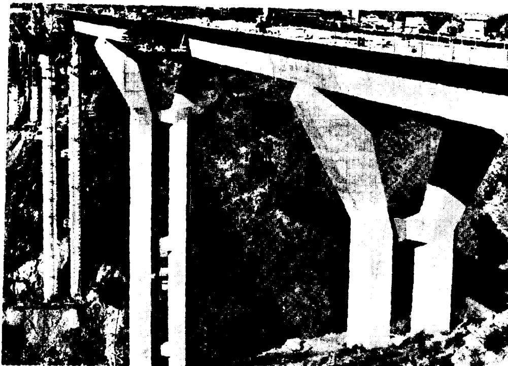
Figure A-23 - Pine Valley Creek Bridge, California
