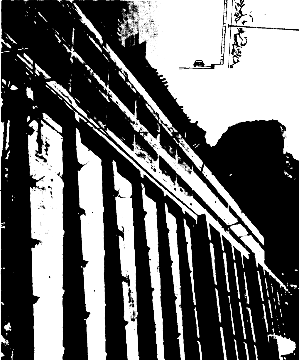
Figure A-13 – Rock face revetment, Switzerland
