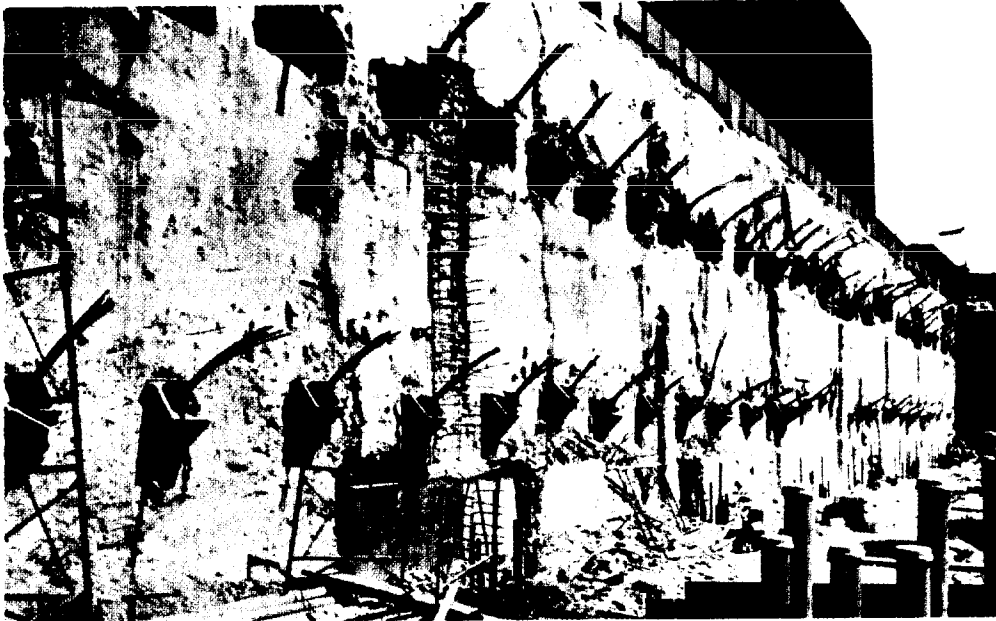
Figure A-3 — Concrete slurry wall. Top level of anchors utilize steel walers to transmit anchor force to wall; bottom layer of anchors use concrete pedestals.
