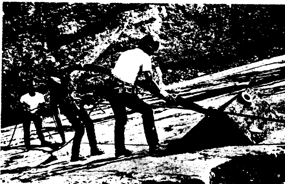
Figure A-16 – Installation of 200 kip anchors, Libby Dam, Montana
