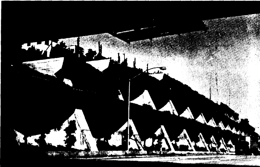
Figure A-6 — Protrero Hill retaining wall, San Francisco
