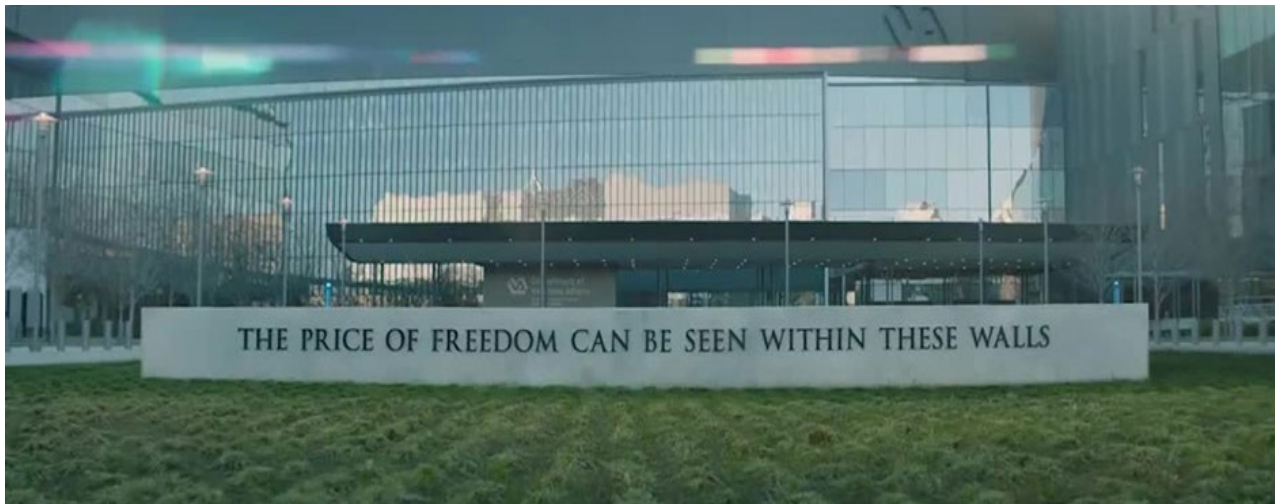
Figure 3. The New Orleans, Louisiana VA Medical Center.
