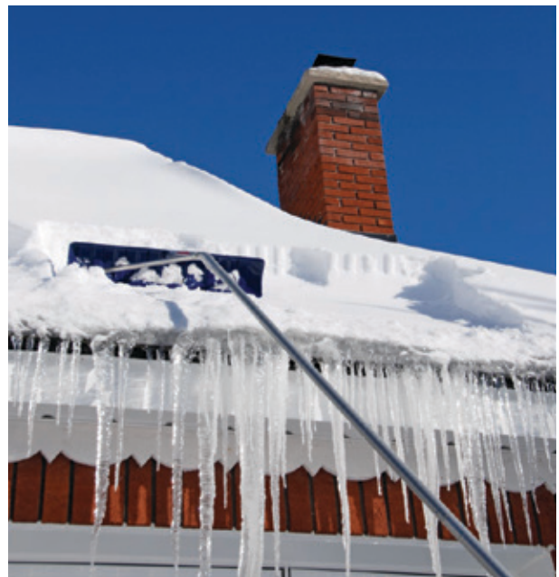
Snow rakes resemble a garden hoe with a long handle. Workers should be instructed to remove small amounts at a time to avoid strain or from being hit or buried by falling snow.
