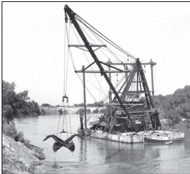
Figure 2-7: Clamshell Dredge Along Sacramento River 1942
