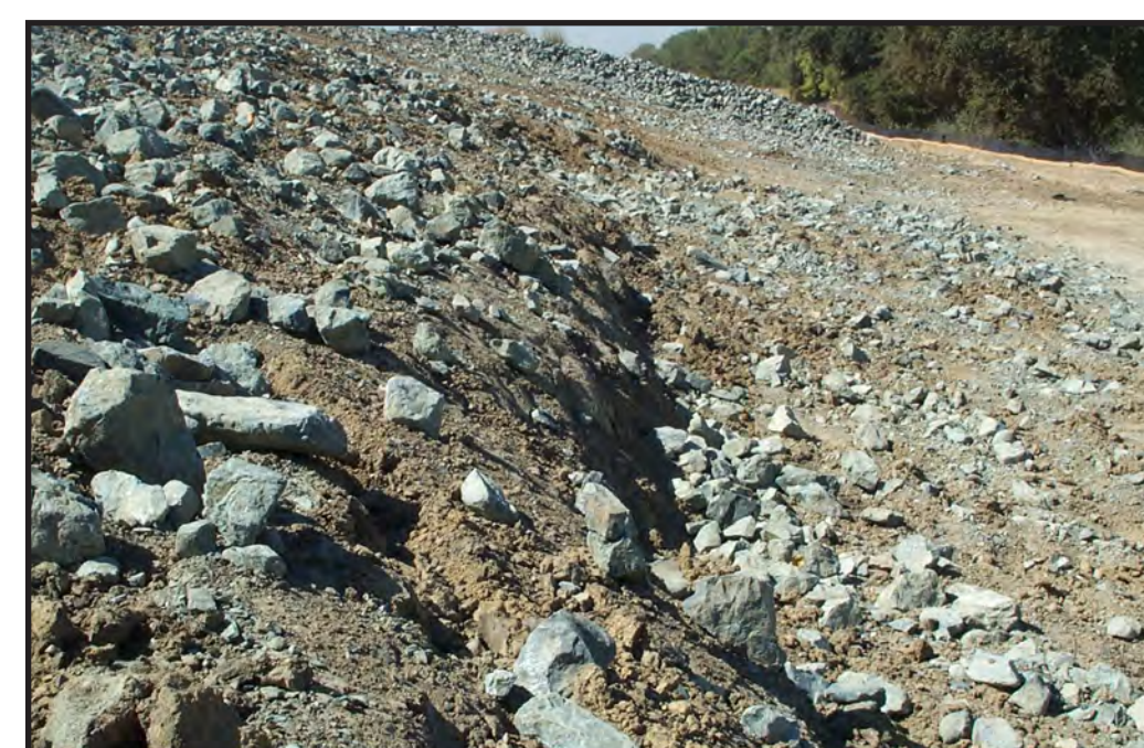
Levee slumping
