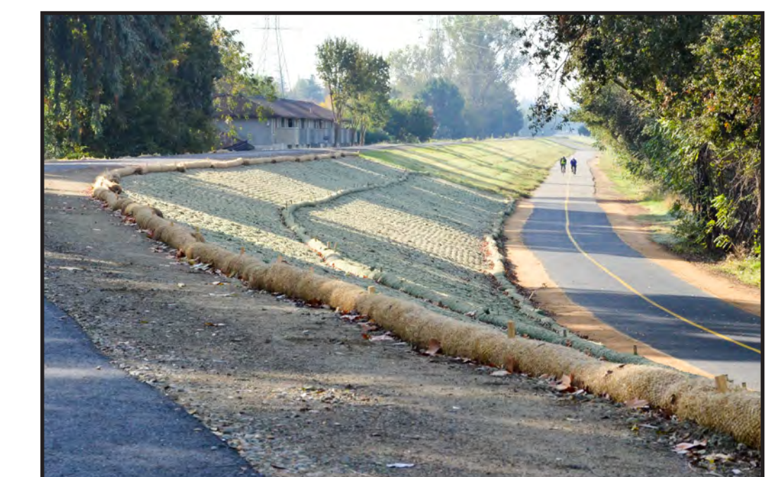
Completed levee with cutoff wall
