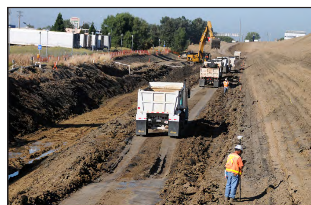
Slump repair
