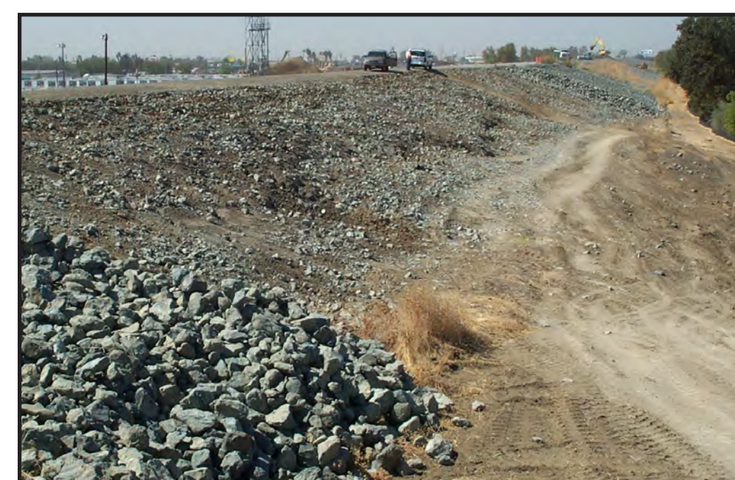
Levee slumping
