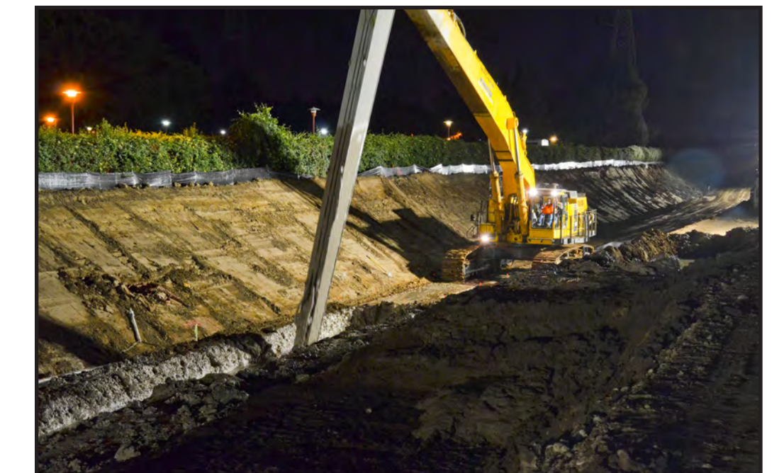
Cutoff wall construction
