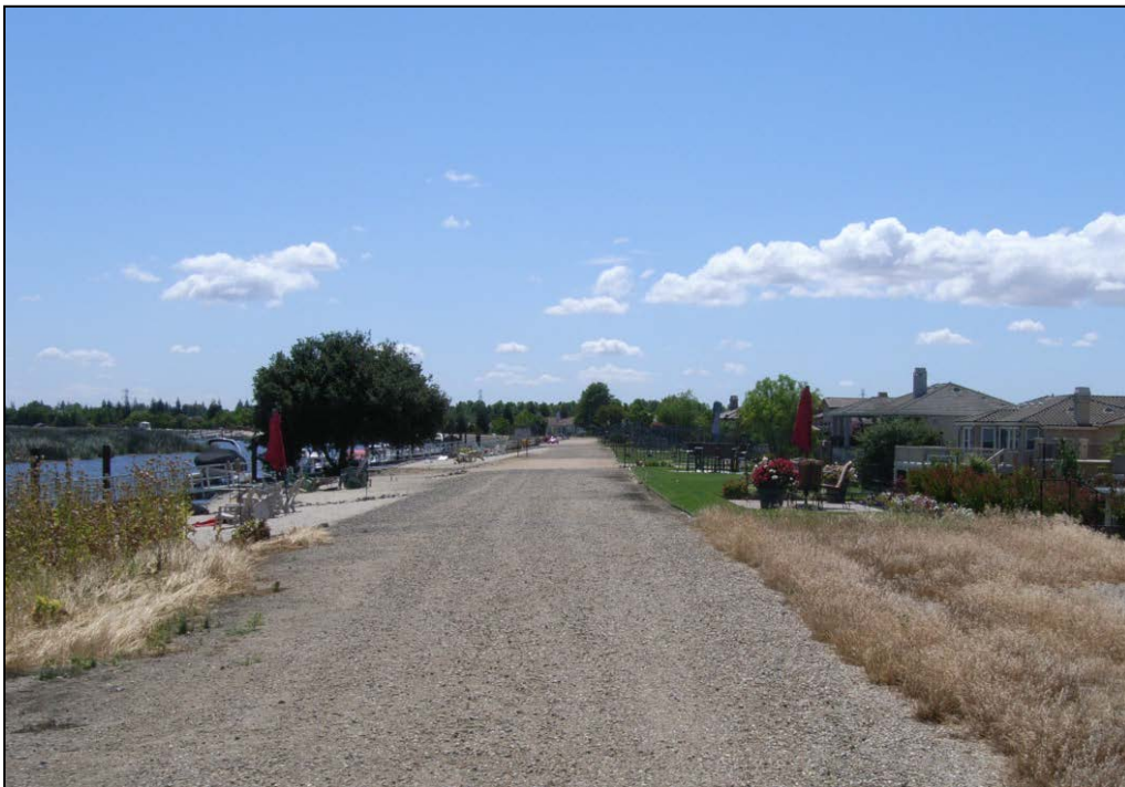
Figure 5-19: Residential Levee with Waterfront Views (Fourteenmile Slough)
