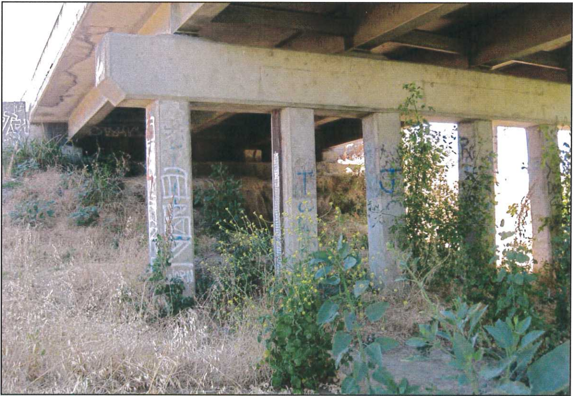
Photo 6. Crows Landing Road Bridge, west side.
