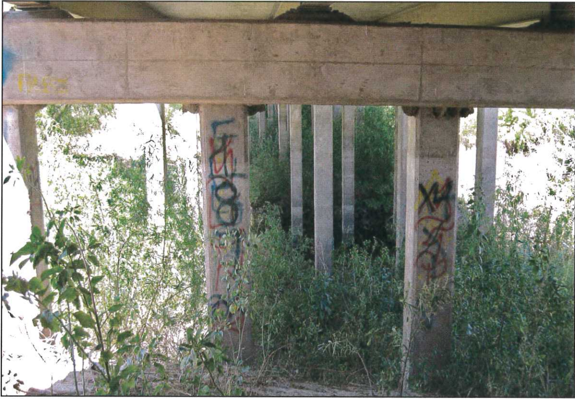
Photo 7. Crows Landing Road Bridge, under west side.
