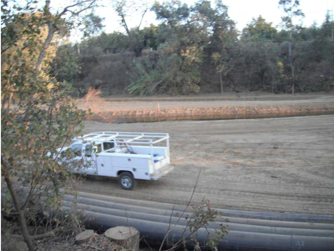
Figure 1: As built floodplain in Phase 1
