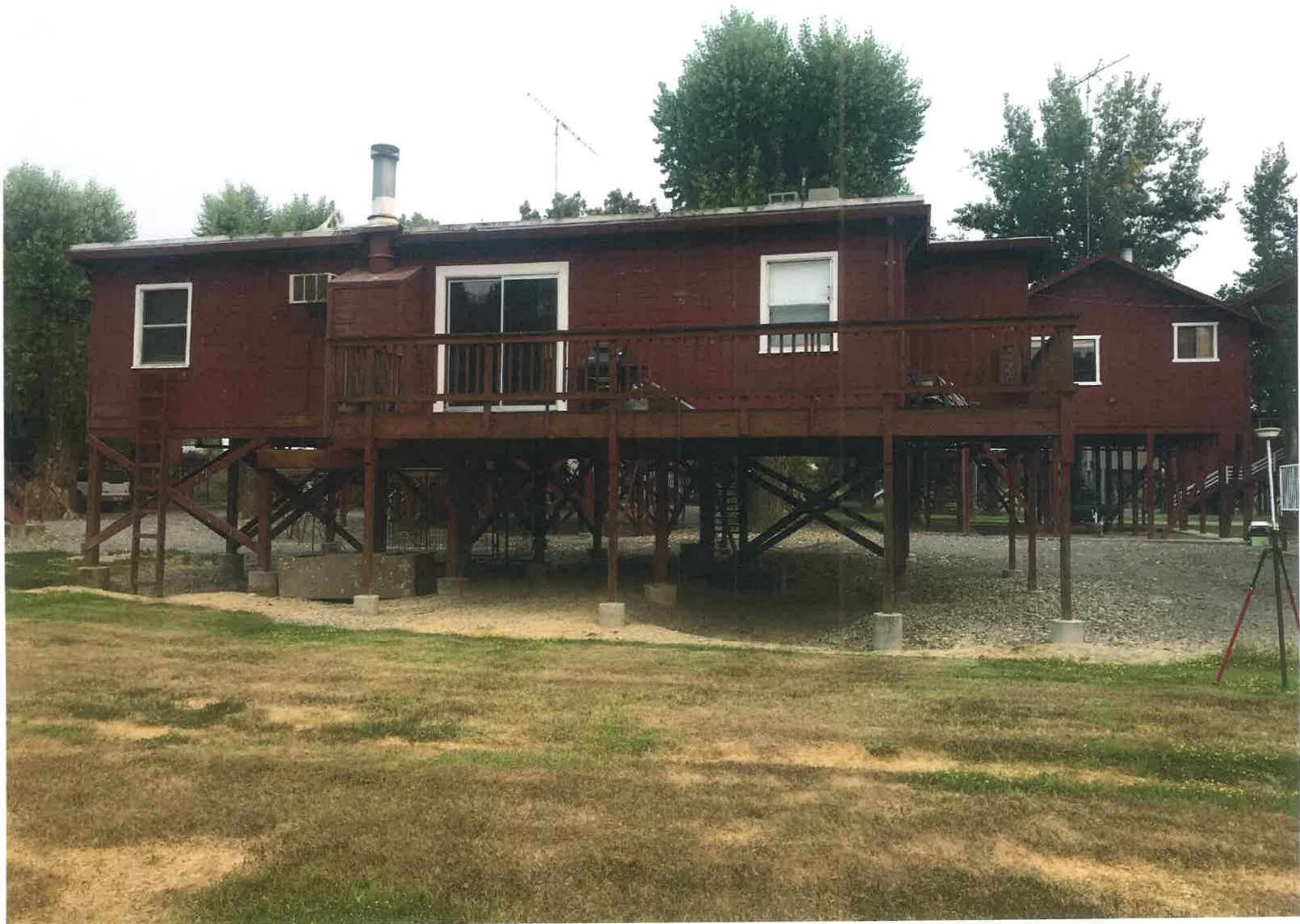
PROJECT SITE VIEW FROM NORTH
