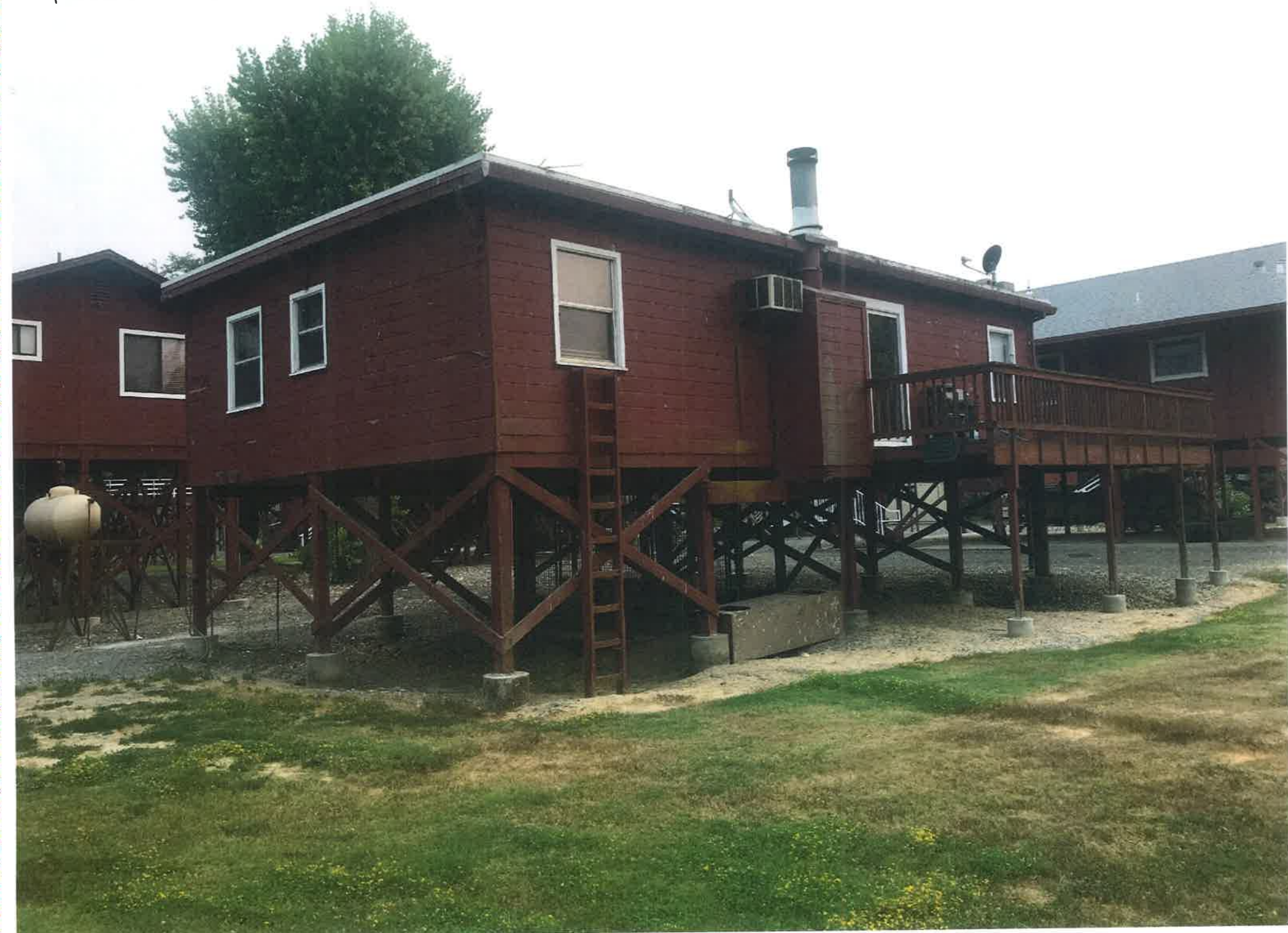
PROJECT SITE VIEW FROM NORTHEAST
