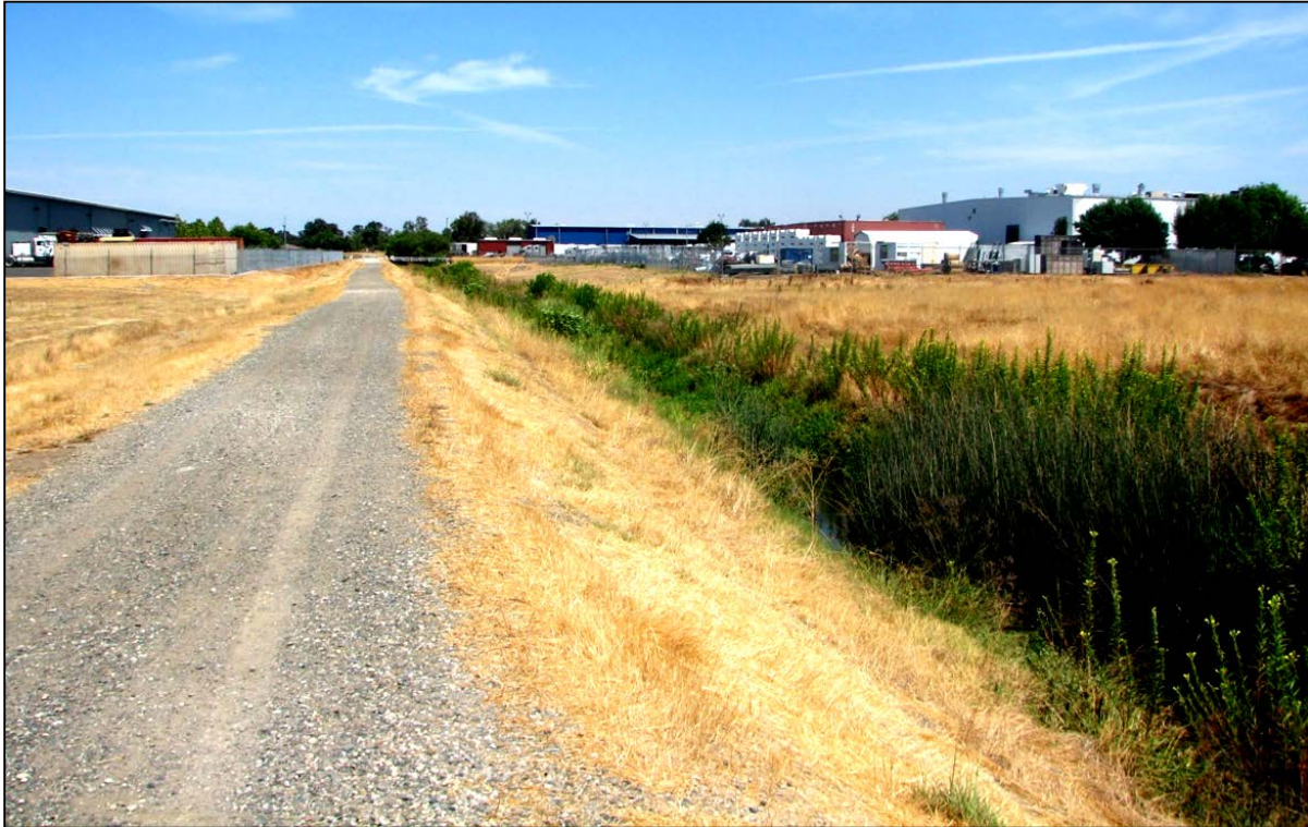
Figure 26. Magpie Creek Diversion Channel.
