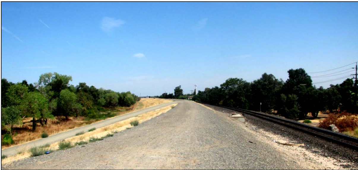
Figure 23. Natomas East Main Drain Canal Levee.
