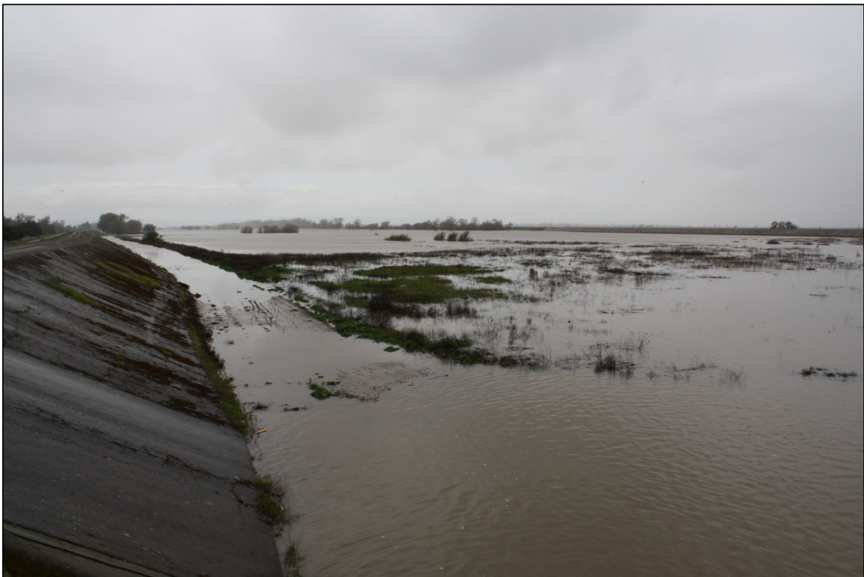
Figure 29. Sacramento Bypass (Downstream of Weir) with Water.
