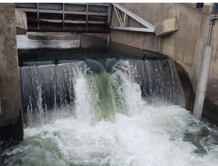
New sluice gate, fully operational, with surface flow for fish passage.
