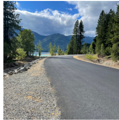
Repaved Boat Launch Road.
