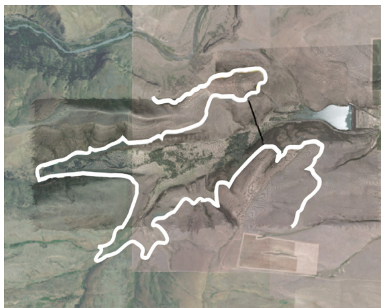
An aerial view of the proposed North Fork Cowiche Creek Reservoir and French Canyon Dam and Reservoir.
