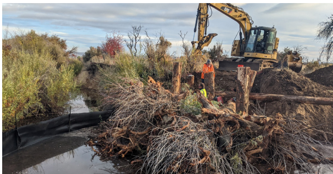
Crews work in Simcoe Creek to add large wood structures.
