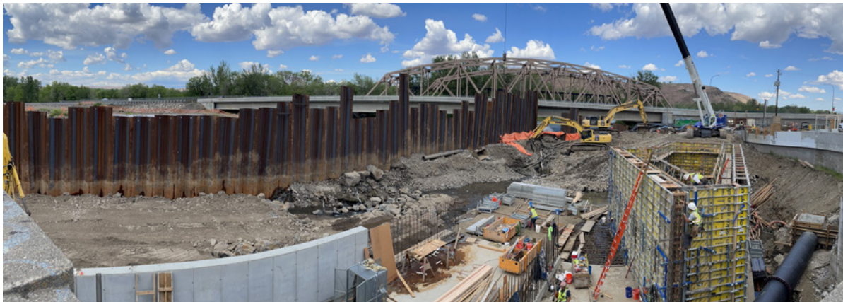
Construction of the city of Yakima's new diversion structure.
