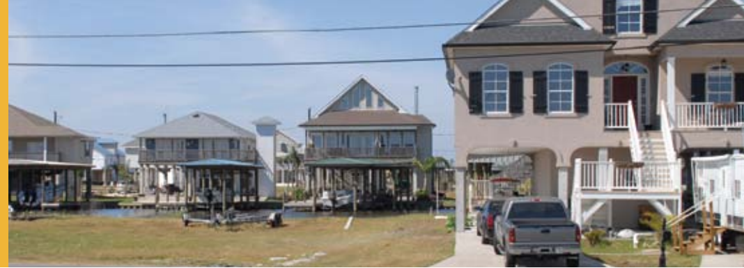
April 4, 2006 — This community in Empire, Louisiana, received no damage from Hurricane Katrina because all homes are built above the floodplain. Marvin Nauman/FEMA
