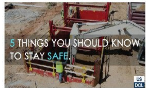
Trench Safety PSA ▶▶
