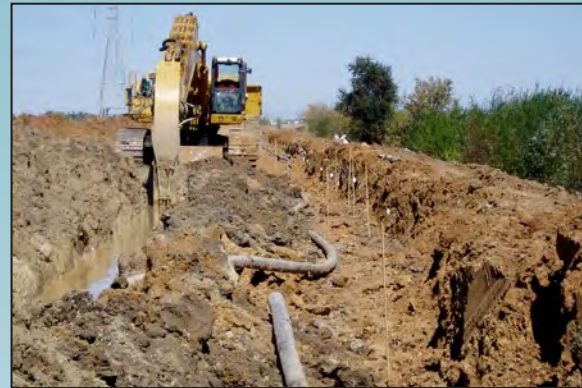
Construction of a slurry cutoff wall
