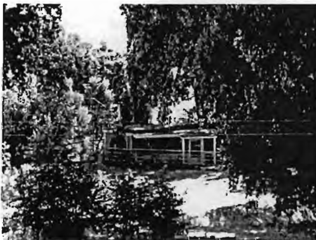
House East of Barn
