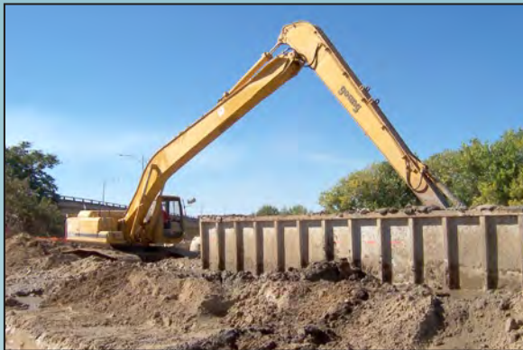
Construction of a slurry cutoff wall
