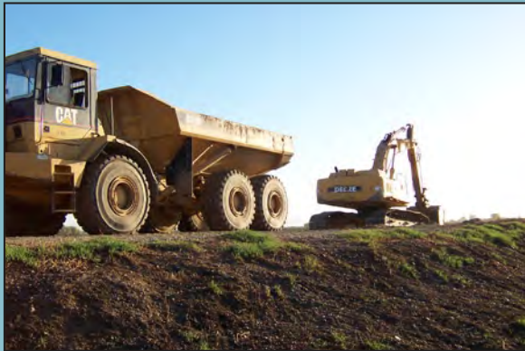
Hauler and excavator on levee crown
