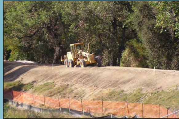
Levee embankment grading
