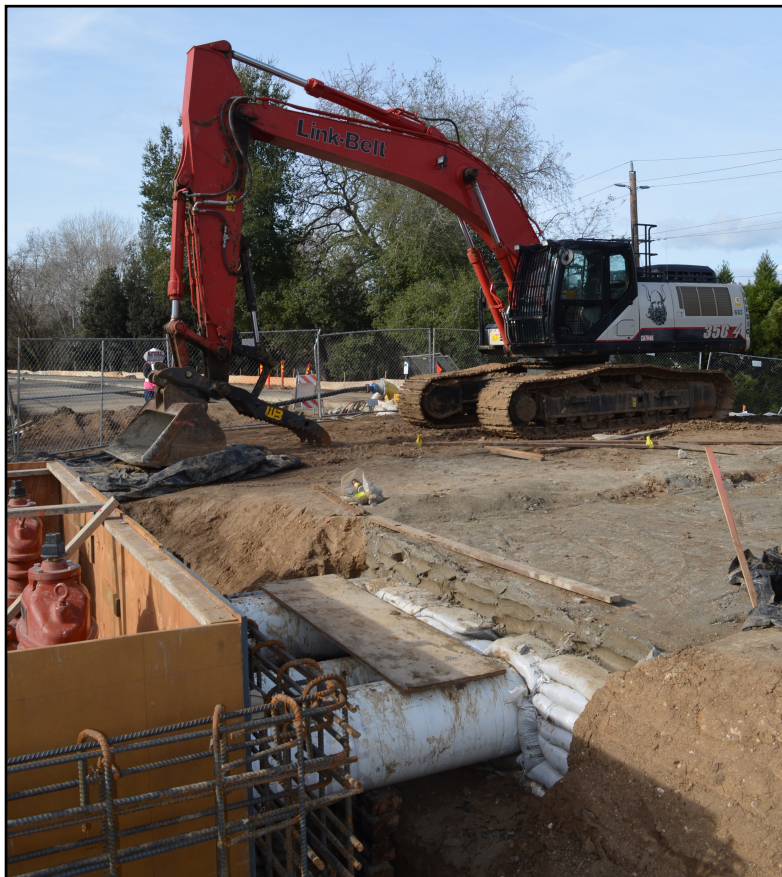
An excavator sits atop Garden Highway as work continues on City of Sacramento Sump 58. Discharge pipes and vault can be seen in the foreground. Sump 58 pumps interior drainage water from the neighborhood to the creek across the roadway.
