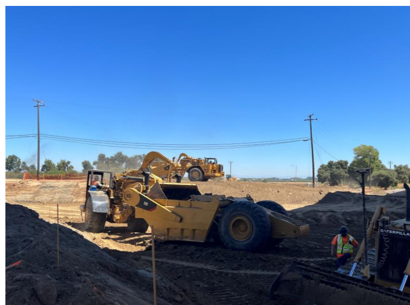
Reach B I-5 Window: Contractor backfilling project site at Interstate 5 cross over
