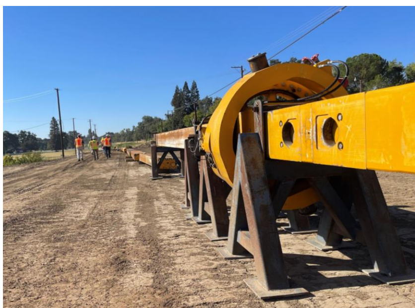
Reach A: Preparing for assembly of the CSM Rig for Cutoff Wall Demonstration Section work at Farm Road
