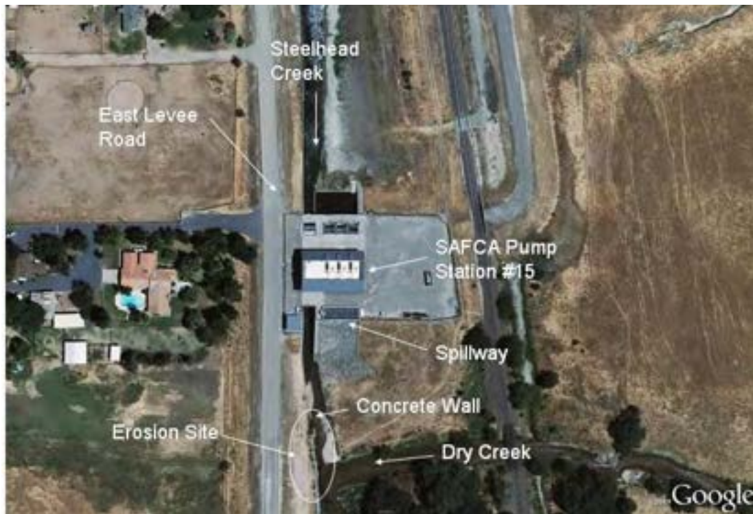
Photograph 1. Aerial imagery of NEMDC erosion site near Dry Creek
