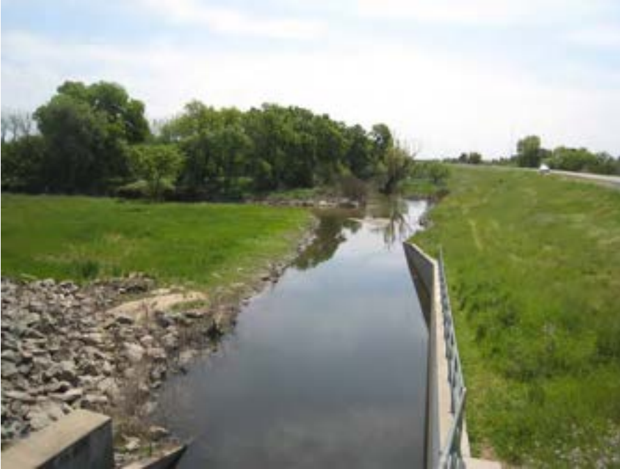
Photograph 2. NEMDC looking downstream from Pump Station 15
