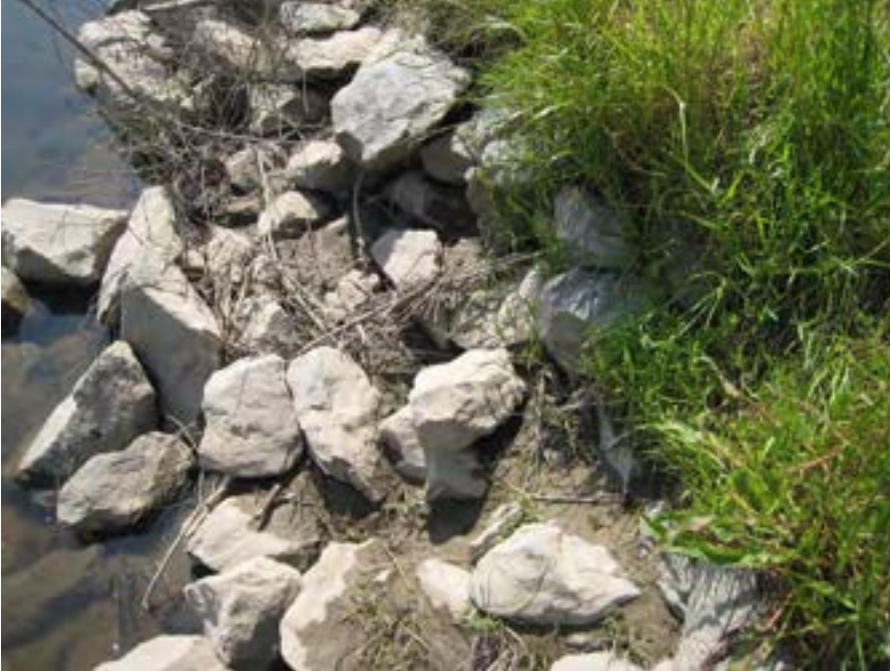
Photograph 4. Rock slope protection along bank
