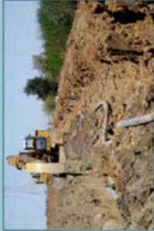
Levee embankment grading
