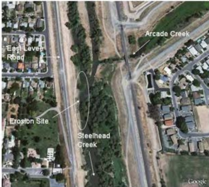
Photograph 5. Aerial view of NEMDC erosion site near Arcade Creek
