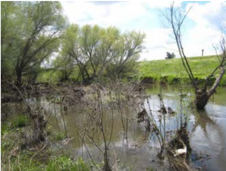
Photograph 6. Erosion along right bank downstream of Arcade Creek
