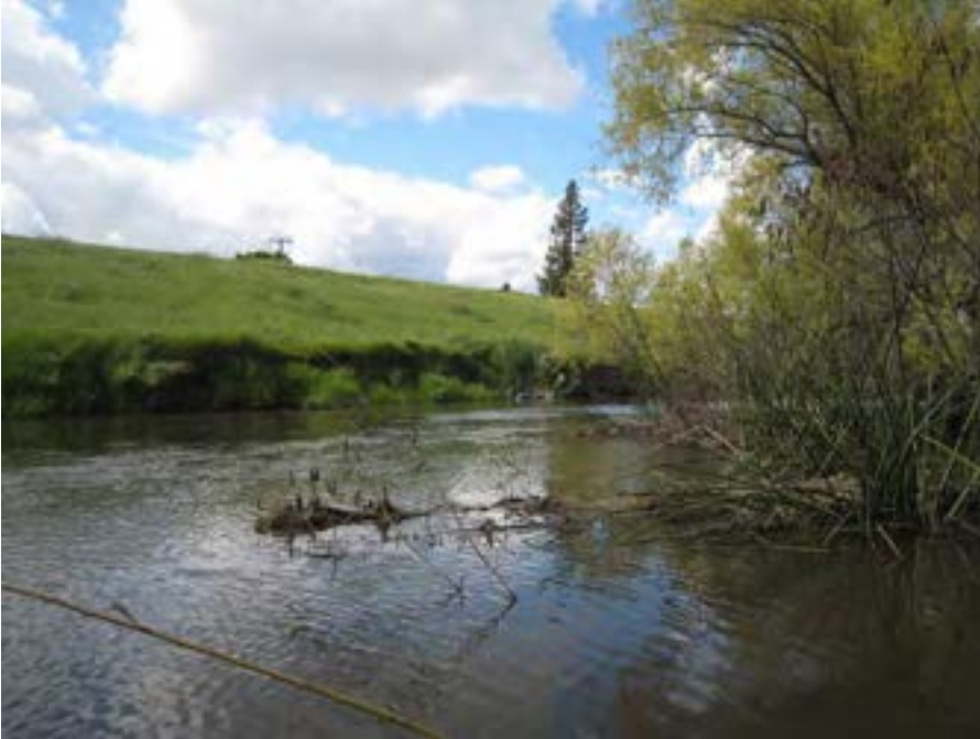
Photograph 7. Erosion along right bank downstream of Arcade Creek
