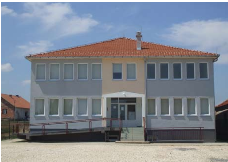
THE NEWLY BUILT COMMUNITY CENTRE IN THE ASHKALI SETTLEMENT OF "DUBRAVĚ/DUBRAVA" IN FERIZAJ/ UROŠEVAC. THE MUNICIPALITY PLANS TO COMPLETE THE INFRASTRUCTURE DEVELOPMENT BY ALSO BUILDING A PLAYGROUND AND A SCHOOL NEARBY.
