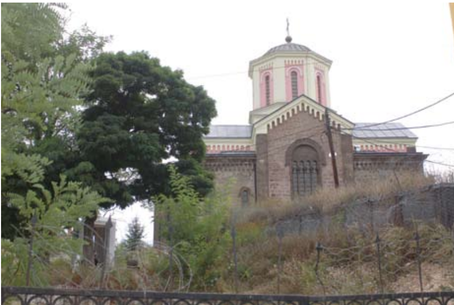
THE SERBIAN ORTHODOX CHURCH OF SVETI (SAINT) SAVA IN SOUTH MITROVICË/MITROVICA, ORIGINALLY BUILT BETWEEN 1896 AND 1912, WAS DESTROYED DURING THE UNREST OF MARCH 2004. ITS RESTORATION BEGAN IN 2007 BY THE COUNCIL OF EUROPE RECONSTRUCTION IMPLEMENTATION COMMISSION ESTABLISHED TO REBUILD RELIGIOUS AND CULTURAL SITES AFFECTED BY THE 2004 EVENTS.
