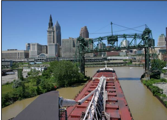
Figure 1.22 - Heading under Eagle Street Bridge
