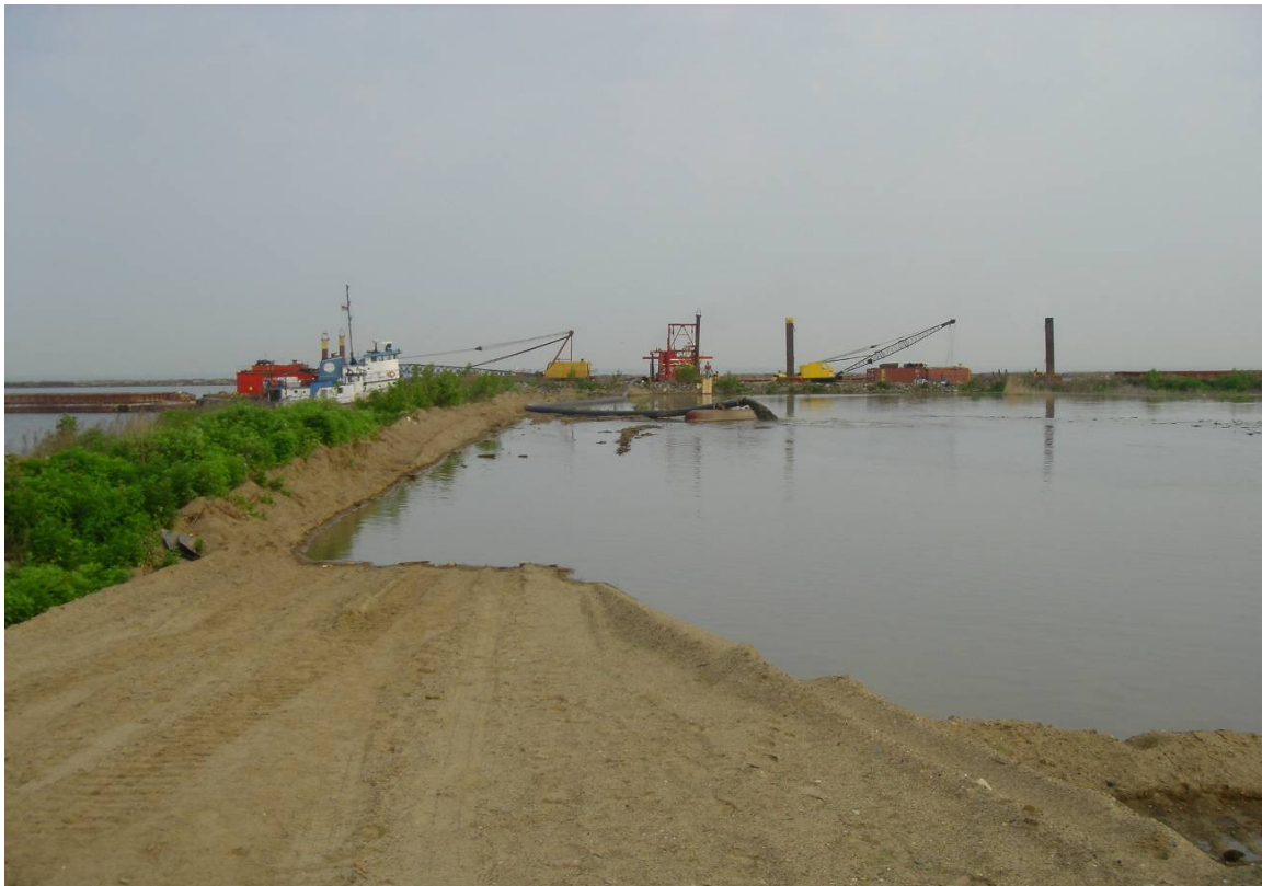
Figure 1.9 – Pumping dredged material from a scow at CDF 10B
