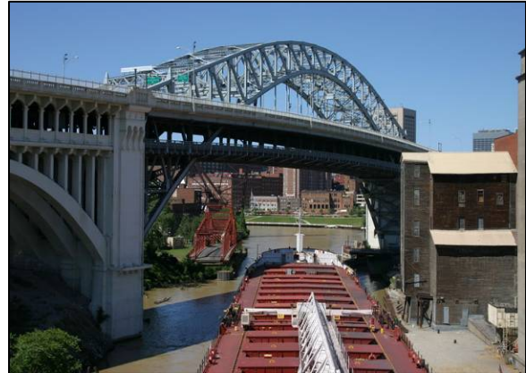
Figure 1.23 - Heading under Veterans Memorial Bridge
