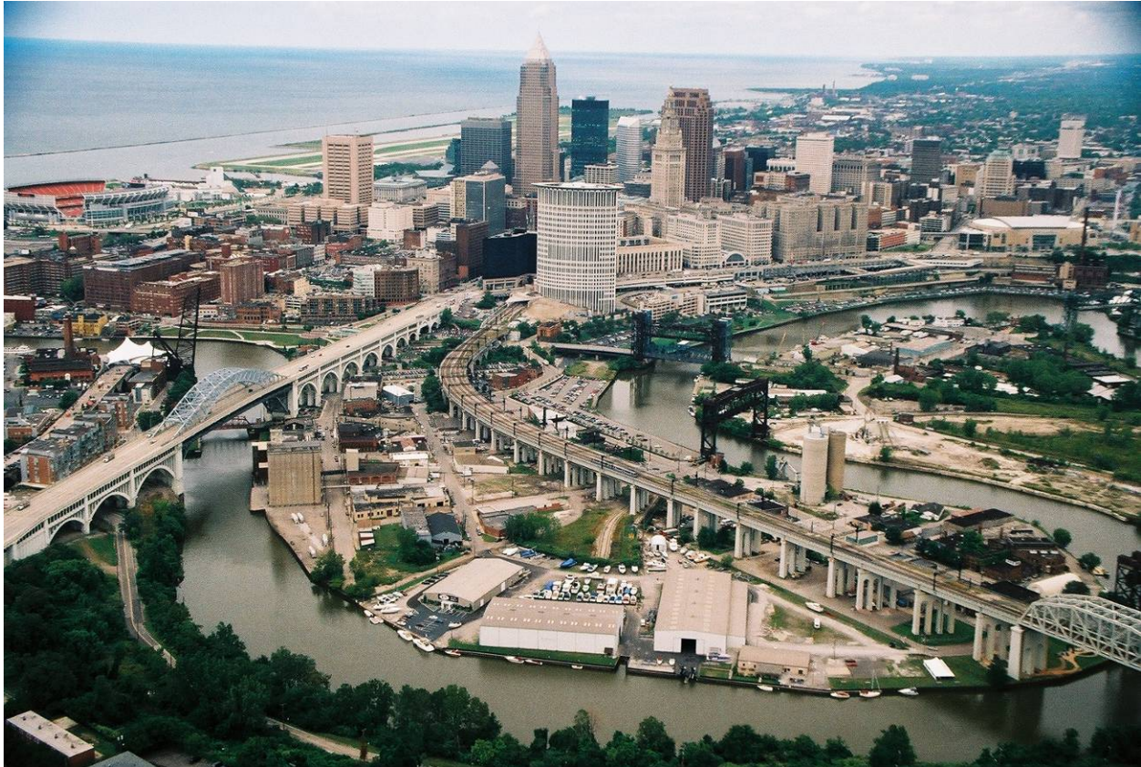
Figure 1.2 – Downtown Cleveland, Ohio
