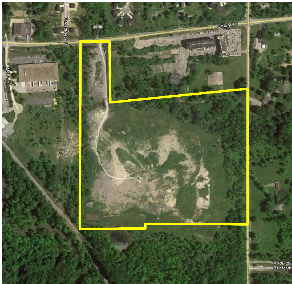
Figure 2-7. Inactive Silver Oak Landfill.
