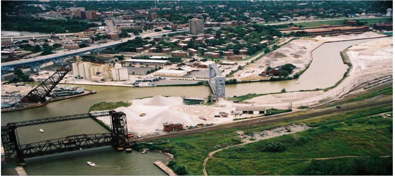
Figure 4. Cleveland Harbor- Inner Harbor-Old River
