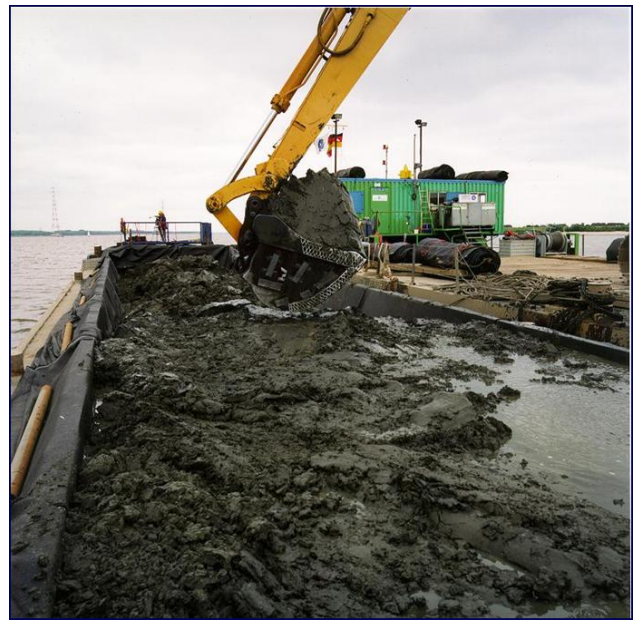
Figure 12 Geocontainer filled with dredged sediment.
