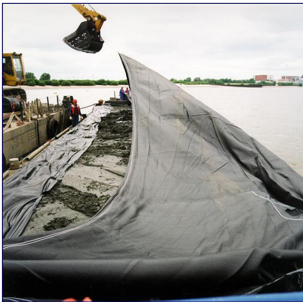
Figure 13 Closing filled Geocontainer.
