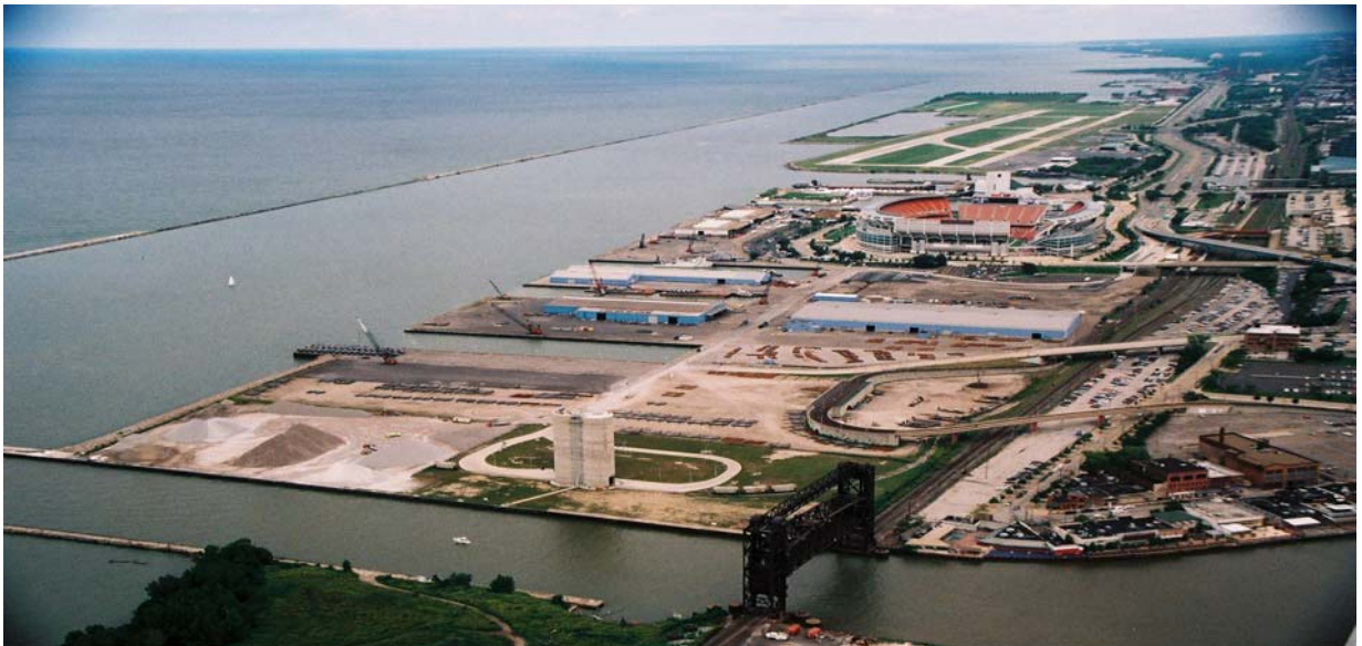
Figure 3- Cleveland Harbor-Outer Harbor- Looking East
