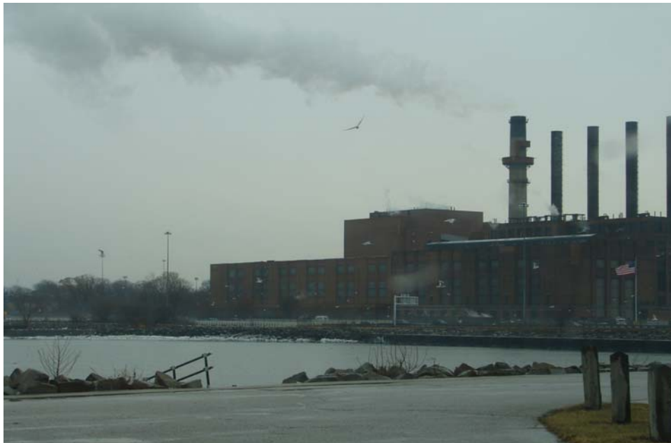
Figure 3. First Energy Power Plant east of Marina. Intake structure is located east of the dike in front of the power plant.
