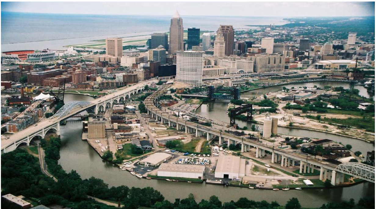
Figure 5-Cleveland Harbor-Inner Harbor-Cuyahoga River
