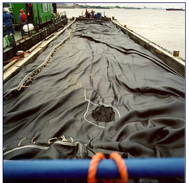
Figure 14 Geocontainer sewn shut.
