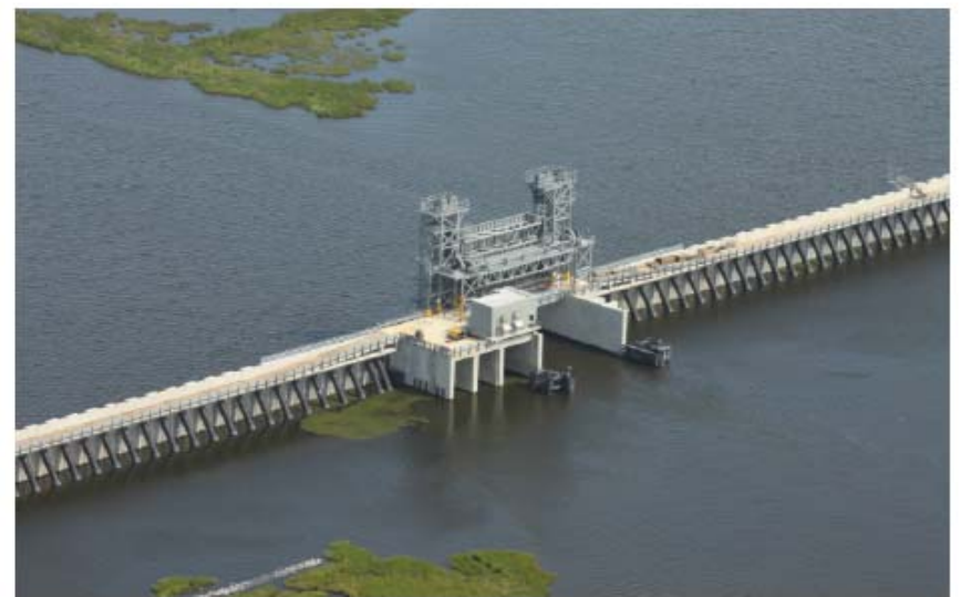
Vertical Lift Gate at Bayou Bienvenue
