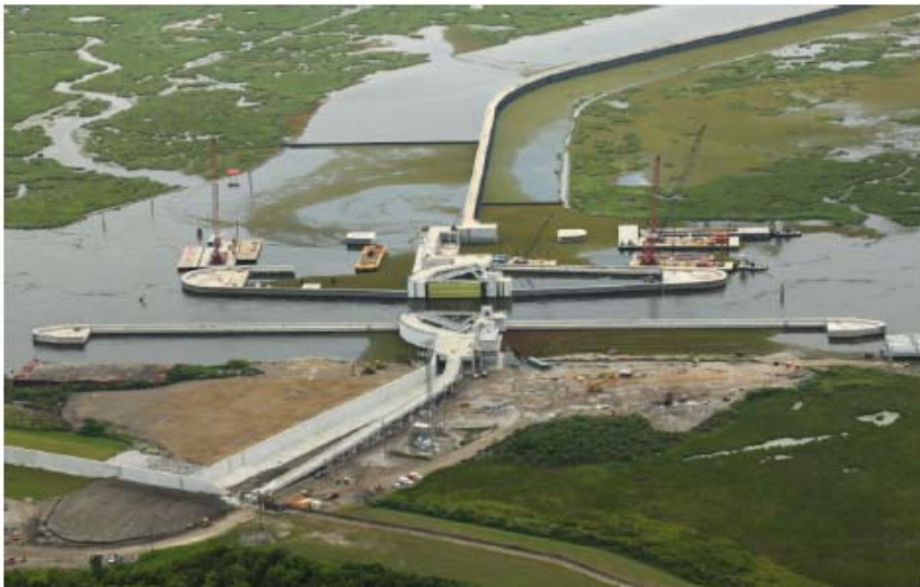
Barge Gate and Sector Gate at the Gulf Intracoastal Waterway
