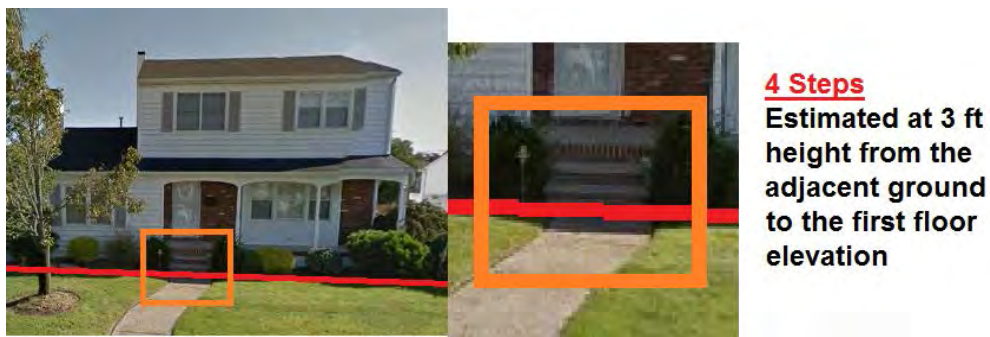
Figure 7. First Floor Elevation
