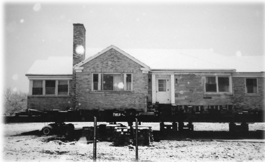
Figure 1. Structure place on a wheels vehicle for relocation to a new site
