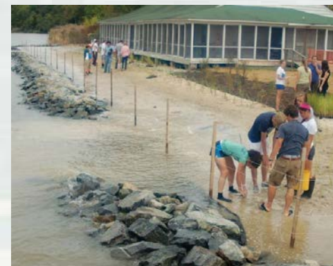
Construction of living shoreline in Camp Pecometh, MD
