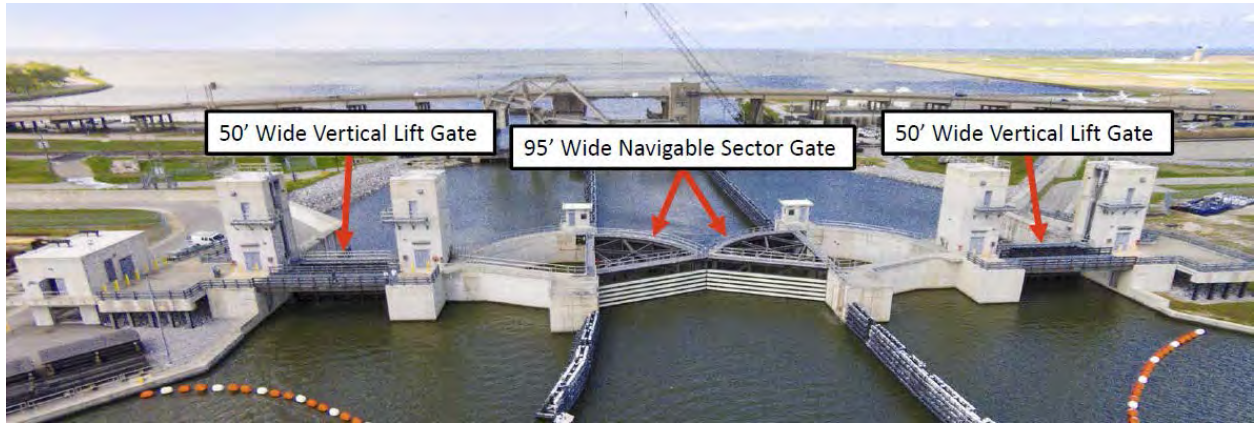
Figure 9-3: Seabrook Floodgate Complex
