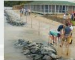
Construction of living shoreline in Camp Peconeth, MD
