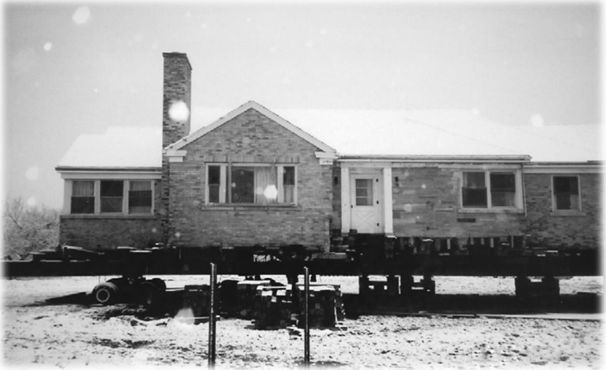
Figure 1: Structure placed on a wheeled vehicle for relocation to a new site
