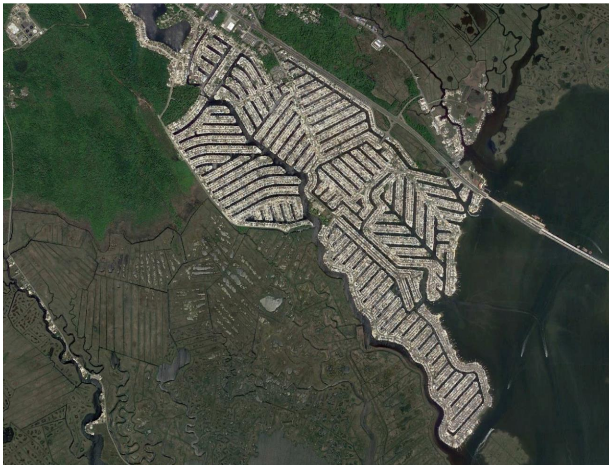
Figure 8: Finger Canal Community Example – Beach Haven West (Stafford Township)
