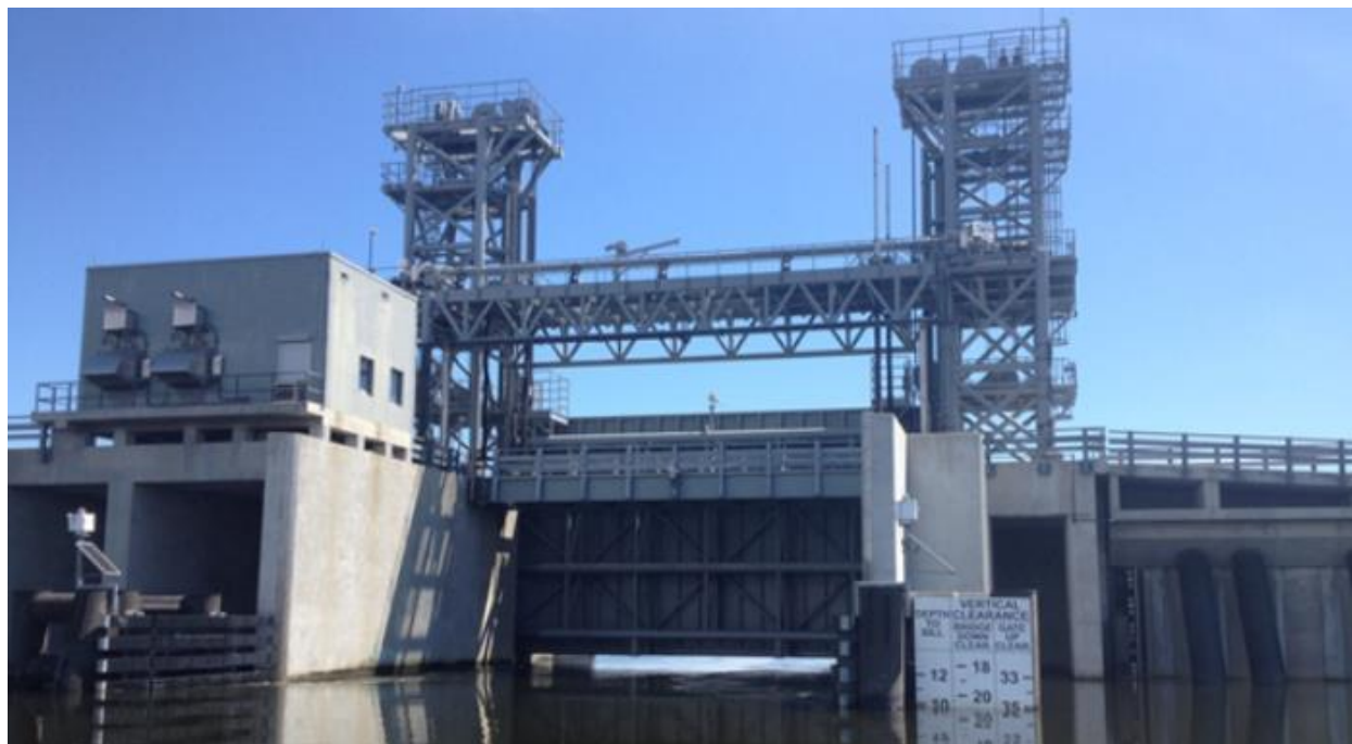
Figure 3-2: Bayou Bienvenue Vertical Lift Gate in New Orleans, LA
