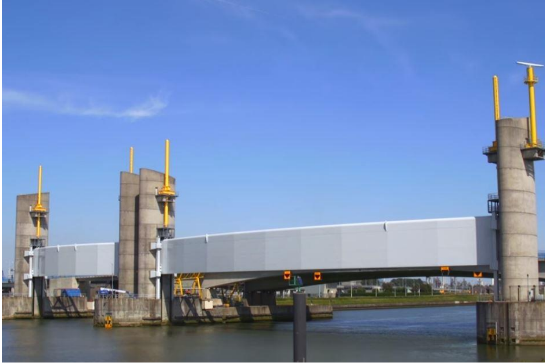
Figure 3-5: Hartel Barrier Vertical Lift Gates
