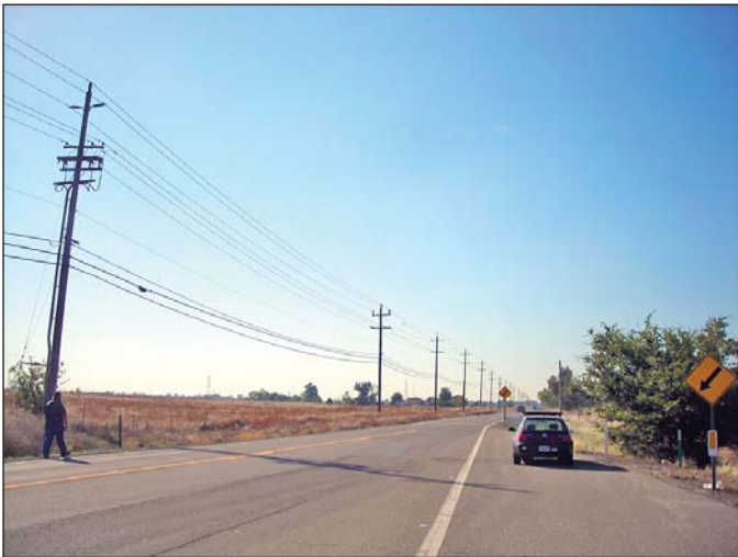
PHOTOGRAPH 2 – Eastern Project site boundary; view to west along Elverta Road.
