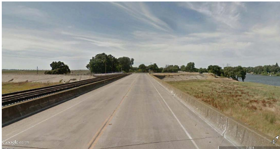
KOP 1: Looking north from Old River Road (on top of the Sacramento Weir). The Sierra Northern Railway railroad tracks, the Sacramento Bypass, and the concrete-lined sides of the Sacramento Weir are visible in the foreground, agricultural fields and the proposed setback levee alignment are in the middleground to the northwest, and the Sacramento River is visible in the middleground to the east. (Google Earth 2016.)
