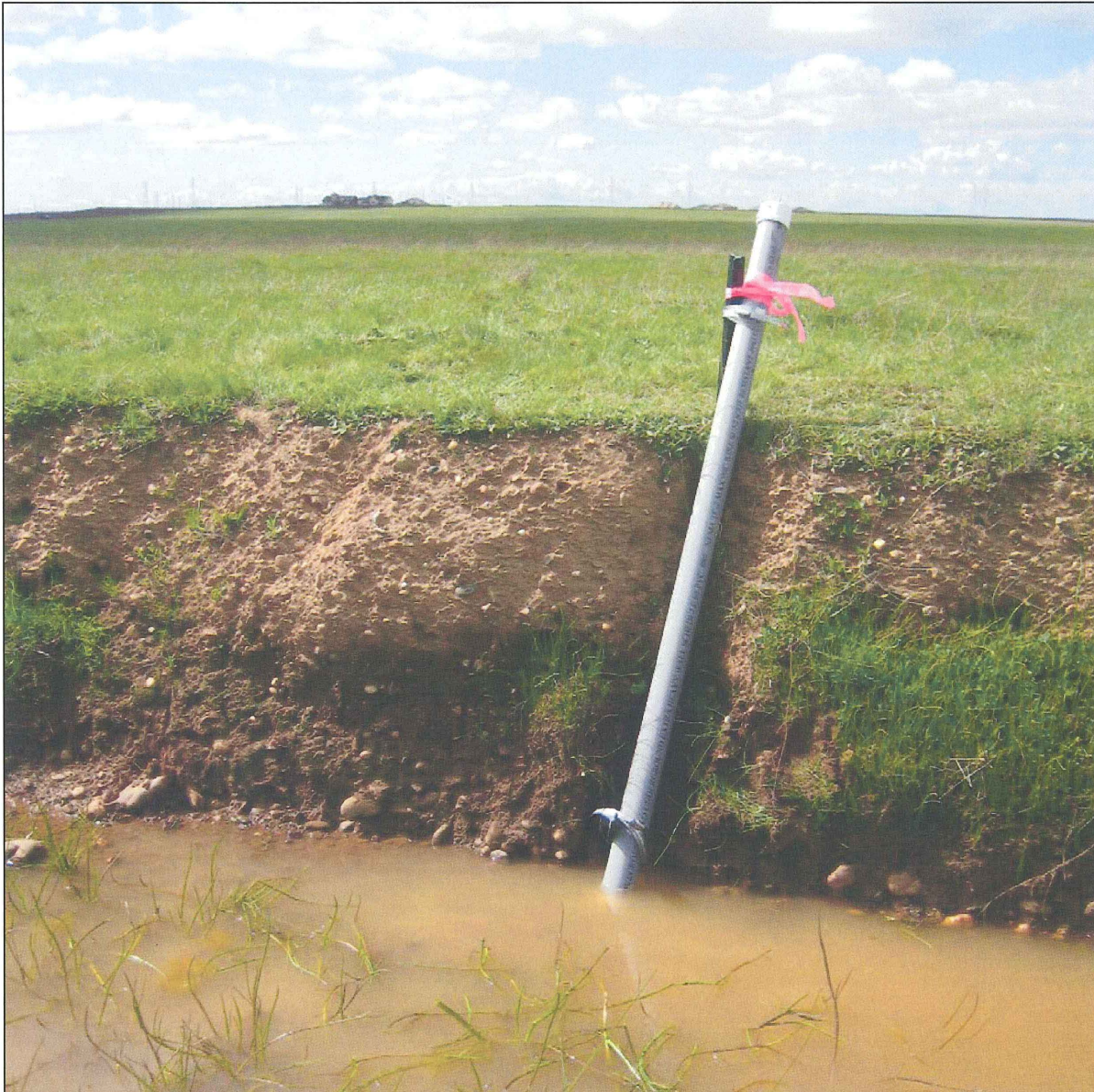
Figure 7. Installation of pressure transducer in stilling well at Klte Creek
