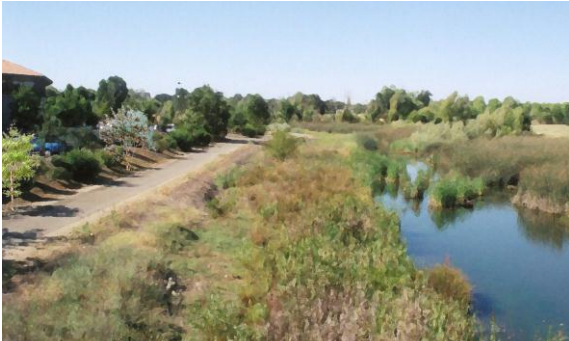
Example of naturalized drainage channel.
