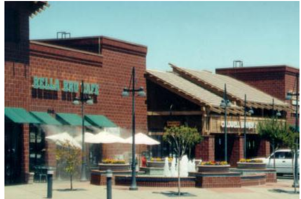
Cornice Detail and Variety of Roof Types
