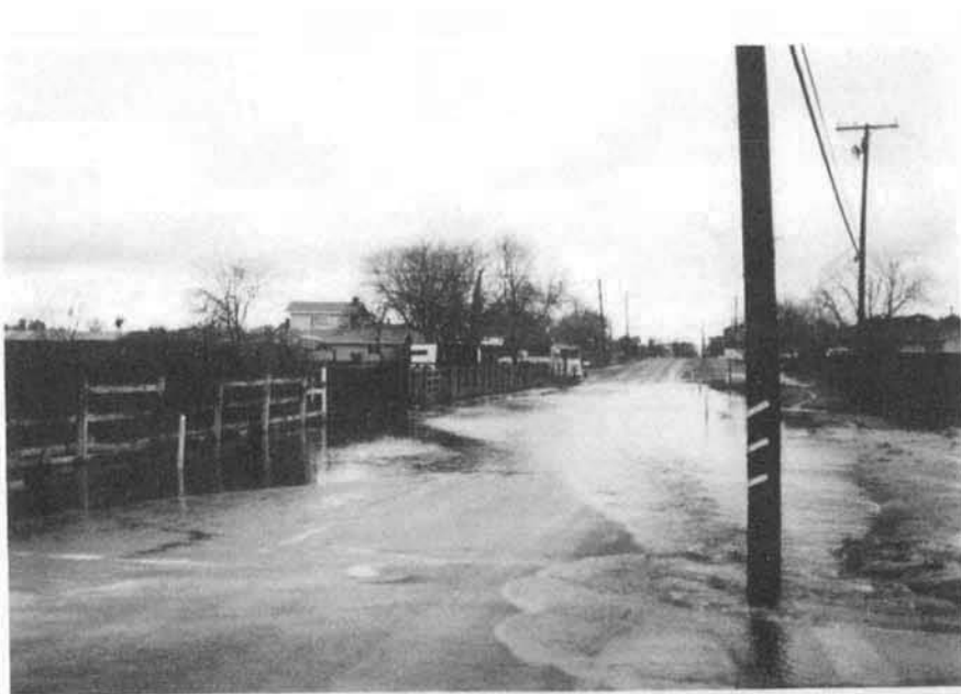
View looking west down U Street at Dry Creek Rd.
