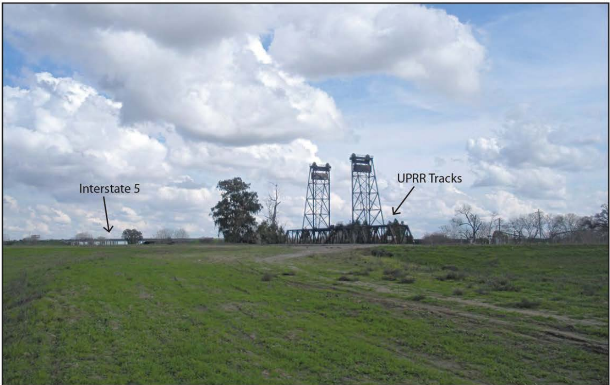
Viewpoint 4. Looking southeast toward UPRR from the action area.
