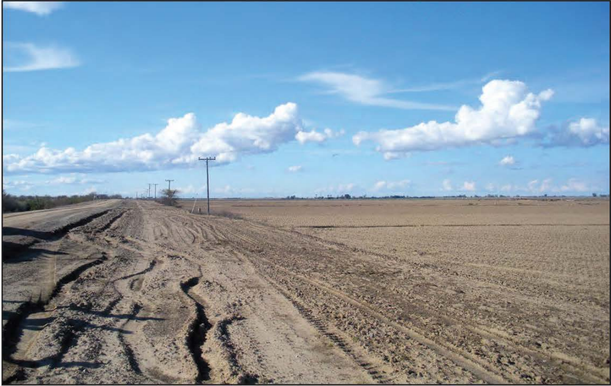
Viewpoint 18. Looking northwest along the Paradise Cut levee (action area at right).
