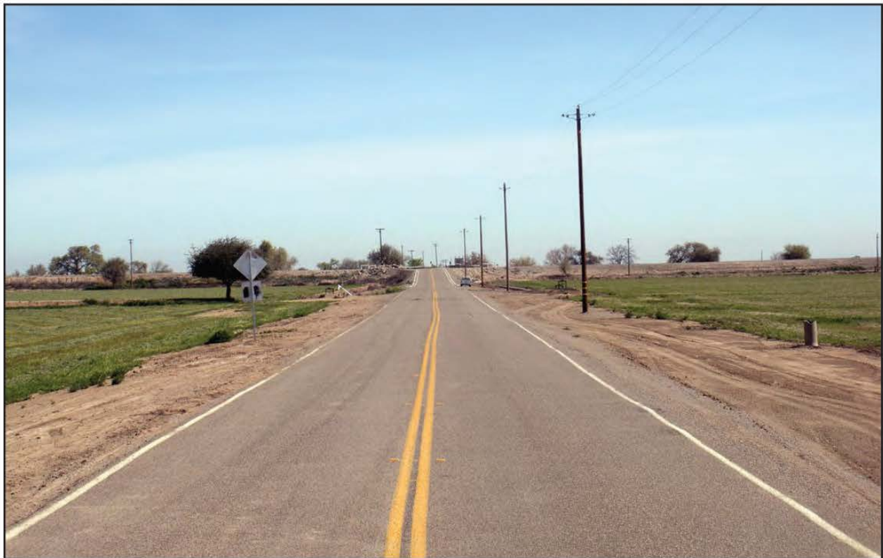
Viewpoint 14. Paradise Road facing northeast toward bridge over Paradise Cut.
