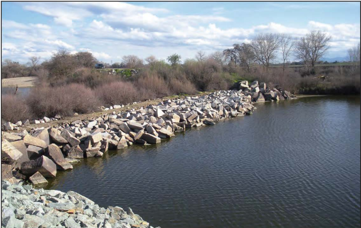
Viewpoint 23. Looking southeast at the Paradise Weir.
