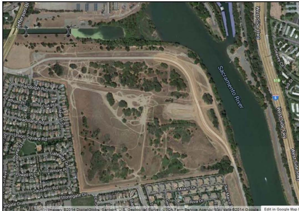
Fig. 4. Construction of the setback levee at the northeast corner of the WSAFCA EIP bordered by the Barge Canal on the north, Sacramento River on the east, and Jefferson Boulevard on the west. Work on the project began on April 6, 2011 and 3 years later, the 2,200 foot long setback levee has not yet been completed. The vacant area in the figure was created on the east by the setback levee, on the north by the barge canal levee, and on the west and south sides by existing levees. Off road vehicles, dirt bikers, paint ballers, hunters, and horseback riders have severely eroded trails into the area that is posted with no trespassing signs. Squatting by homeless people and illegal dumping is common. The closure of the South River Road to construct the setback levee has created a haven for drug dealers and crime due to isolation caused by the absence of regular traffic. An intent of the setback levee project was preservation of wildlife habitat, but few desirable native plants and wildlife find sanctuary in the vicinity.
