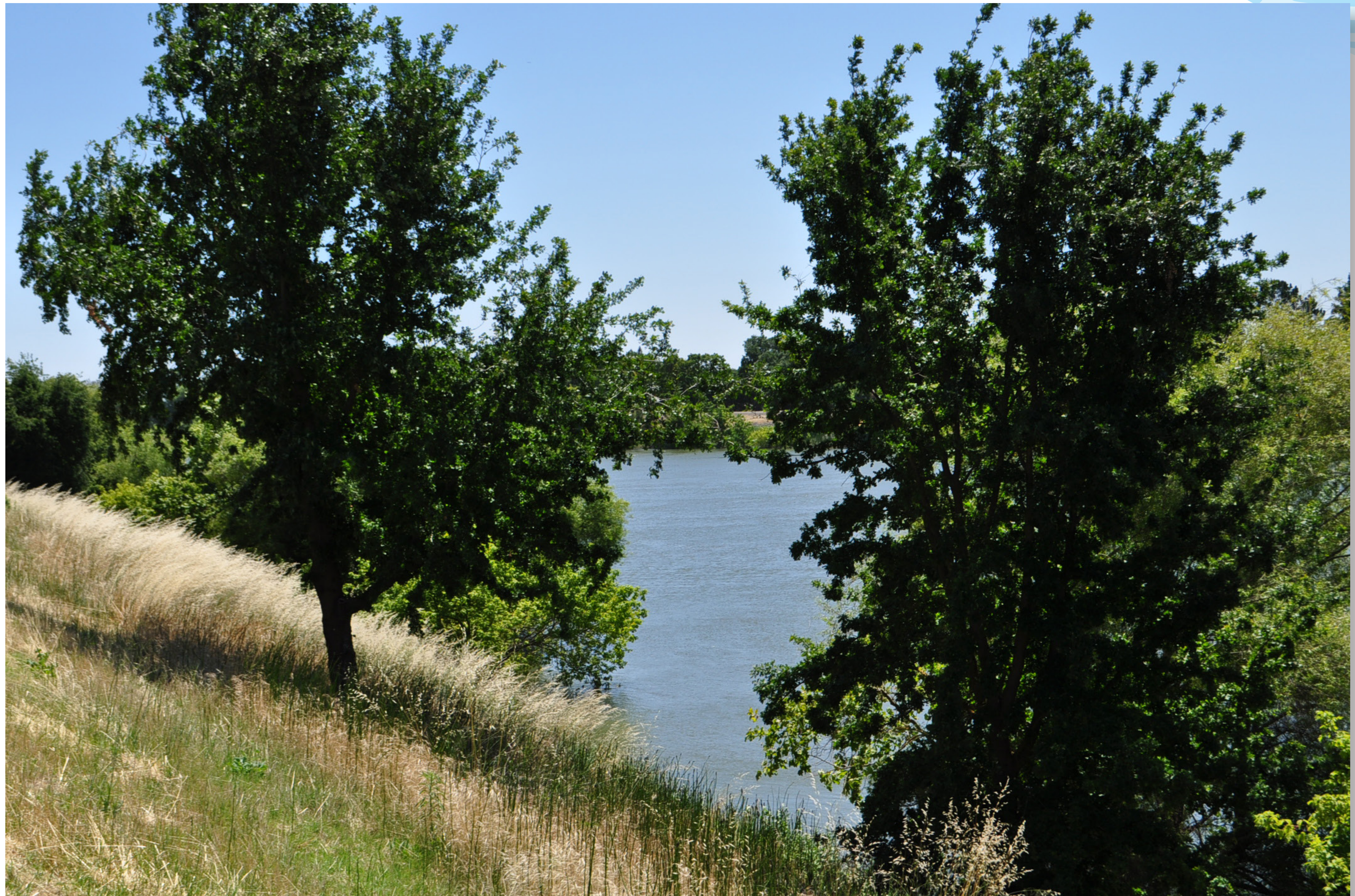
On South River Road, looking east and across the river toward Sacramento's Little Pocket neighborhood. This levee stretch is included in the 6 miles proposed for upgrades under the Southport Sacramento River EIP.
