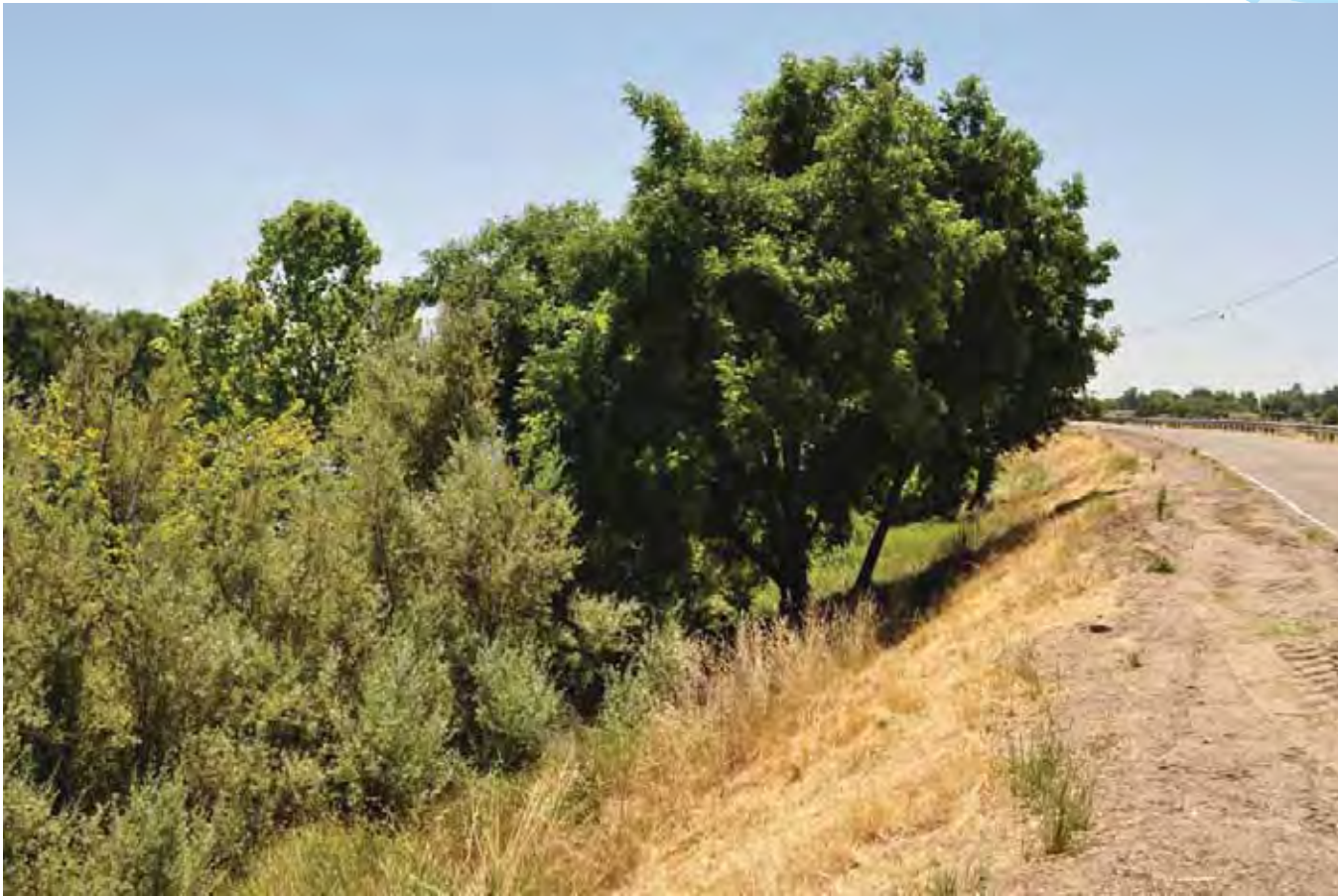
South of Davis Road on South River Road looking southeast at the waterside slope of the levee, on which the Southport Sacramento River EIP is proposed to be implemented.
