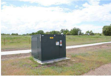
Figure 2 – Capacitor Bank
