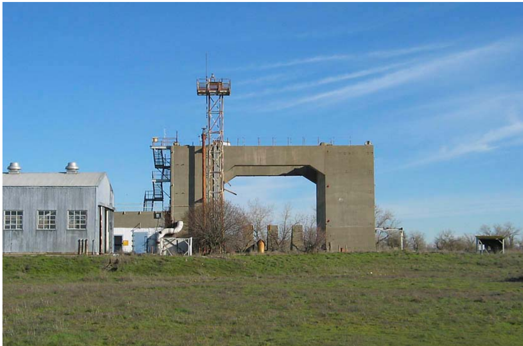
Viewpoint 2 – This view of an abandoned rocket testing facility was taken from the southern portion of the project site looking north. All aerospace facilities would be removed prior to project construction activities.
