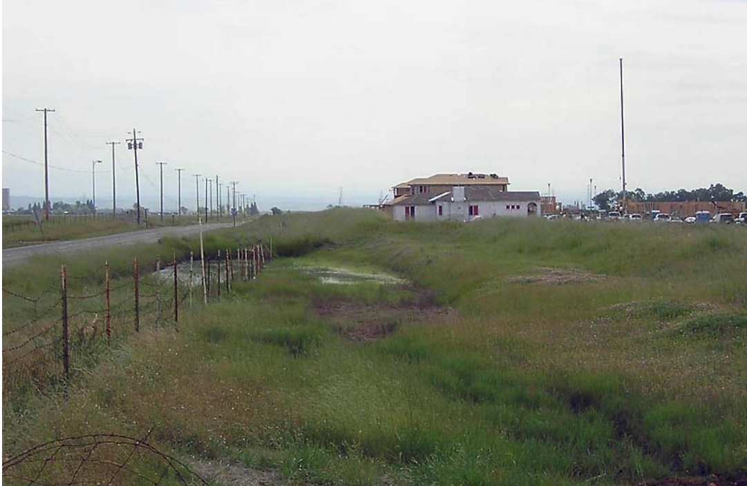
Viewpoint 7 – Views from the southern portion of the project site include the approved Sunrise Douglas Community Plan area, located south of Douglas Road. Shown here are new homes under construction in the Anatolia Phase 1 development.
