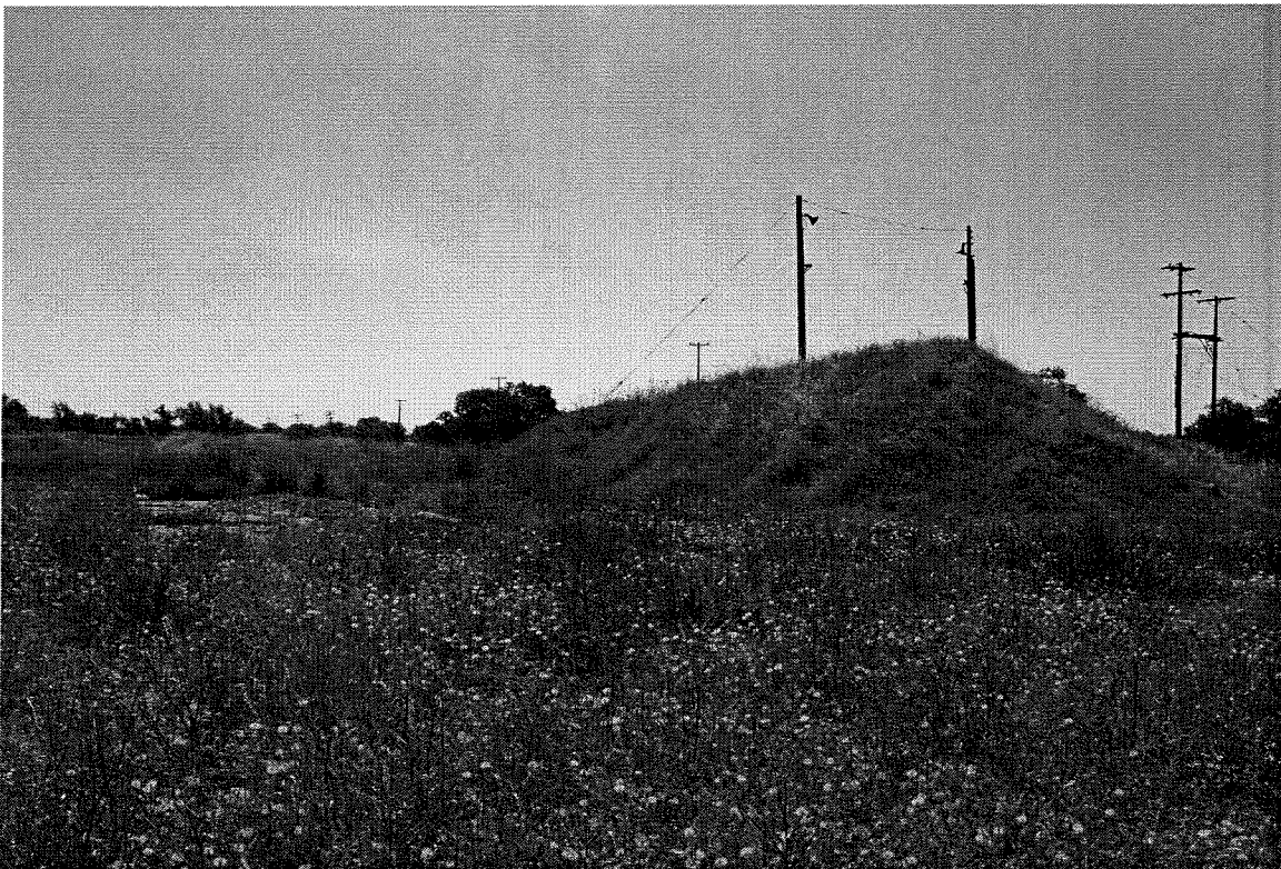
Plate 44: Destruct Pad, bracketed to the south by the earthen berm of the original test site, Sigma Test Area, 1961. Looking east/southeast. View of May 2005.
