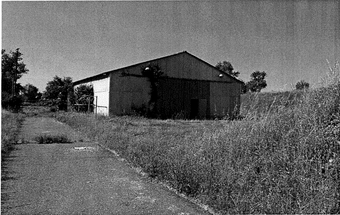
Plate 18: Motor Storage Building (Unit 104), Solid Propellant Assembly Area, 1956. Looking south/southwest. View of May 2005.
