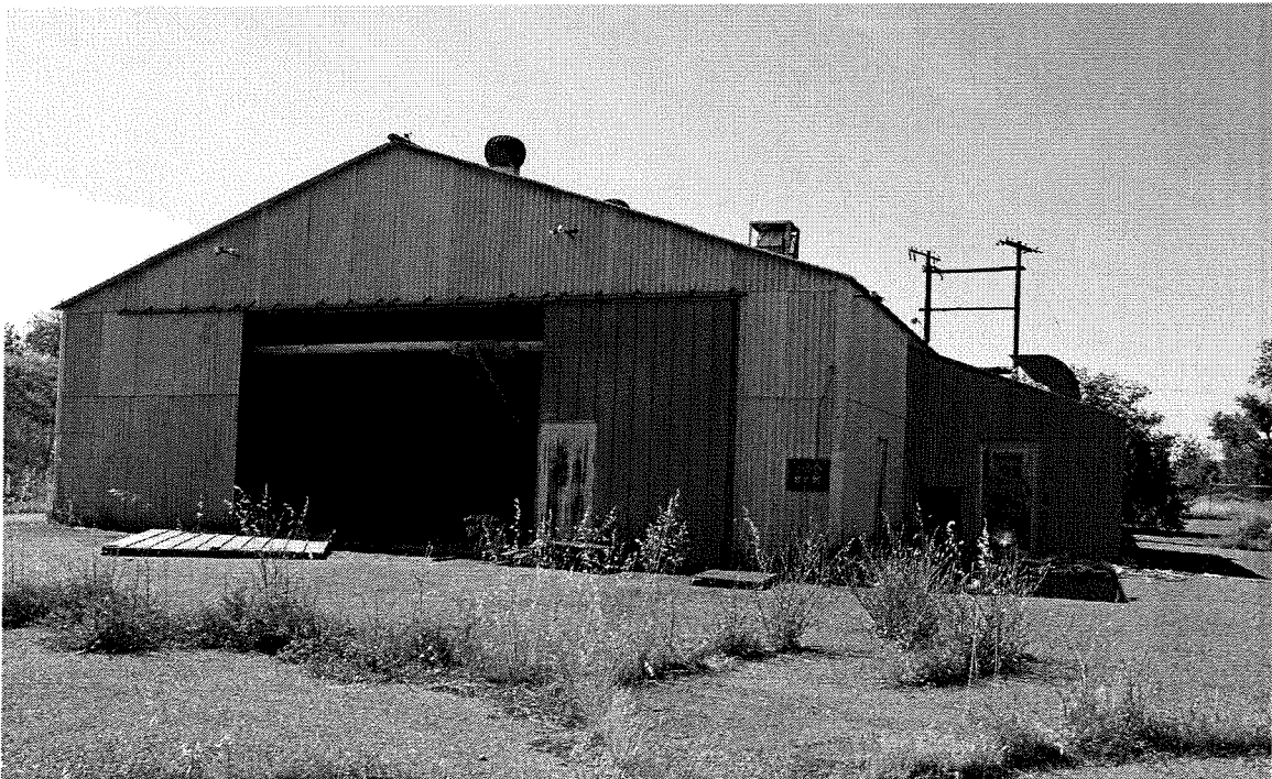
Plate 22: Assembly Building (Unit 103), Solid Propellant Assembly Area, 1956. Looking south/southeast. View of May 2005.
