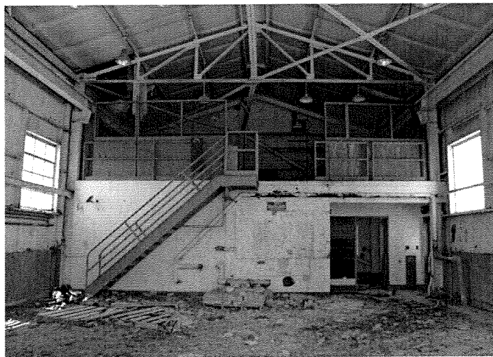
Plate 113: Shop for Test Stand No. 3 (Unit 133), Beta Test Complex, 1963-1964. Interior. Looking west. View of May 2005.
