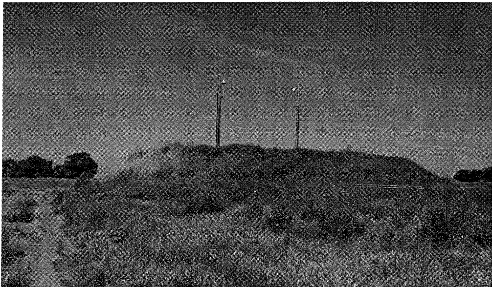
Plate 41: Test Area and Support Building (Unit 95), surrounded by earthen berm, Sigma Test Area, 1956-1961. Looking west. View of May 2005.
