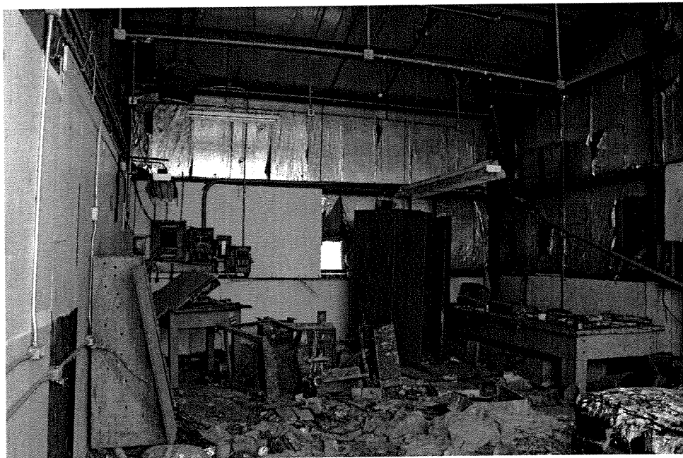
Plate 75: Generator-Compressor Building (Unit 62), Alpha Test Complex, 1956-1957. Interior. View of May 2005.
