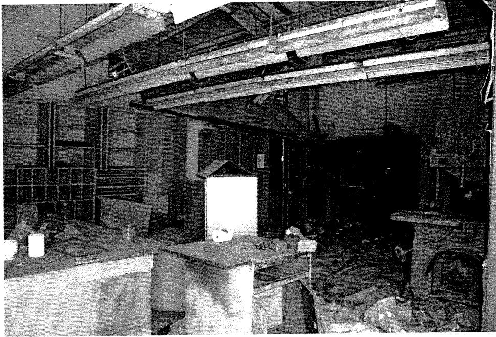
Plate 74: Generator-Compressor Building (Unit 62), Alpha Test Complex, 1956-1957. Interior. View of May 2005.
