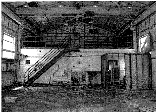
Plate 143: Shop for Test Stand No. 1 (Unit 124), Beta Test Complex, 1963-1964. Interior. Looking northwest. View of May 2005.
