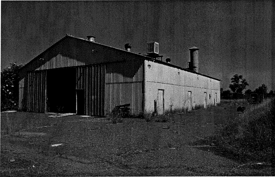
Plate 21: Assembly Building (Unit 103), Solid Propellant Assembly Area, 1956. Looking northwest. View of May 2005.
