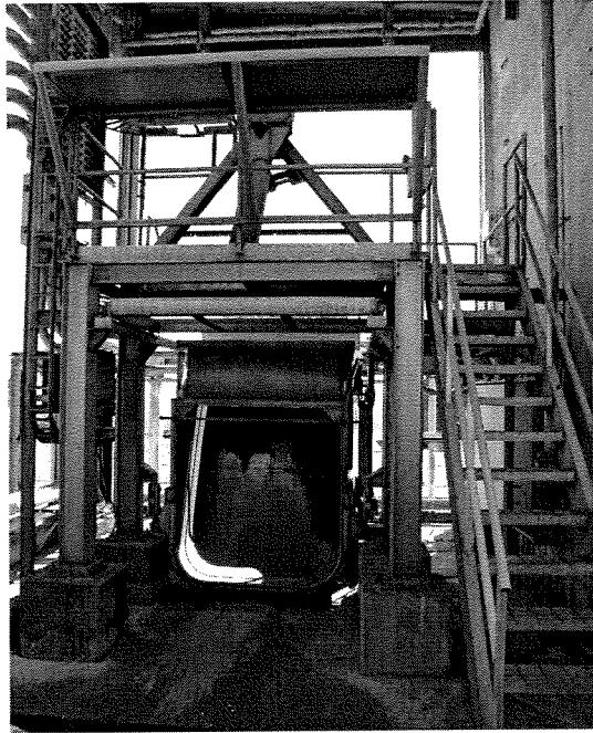
Plate 155: Test Structure (Unit 32), Gamma Test Area, 1964. East test cell, with scaled captive firing stand intact. Looking northwest. View of May 2005.
