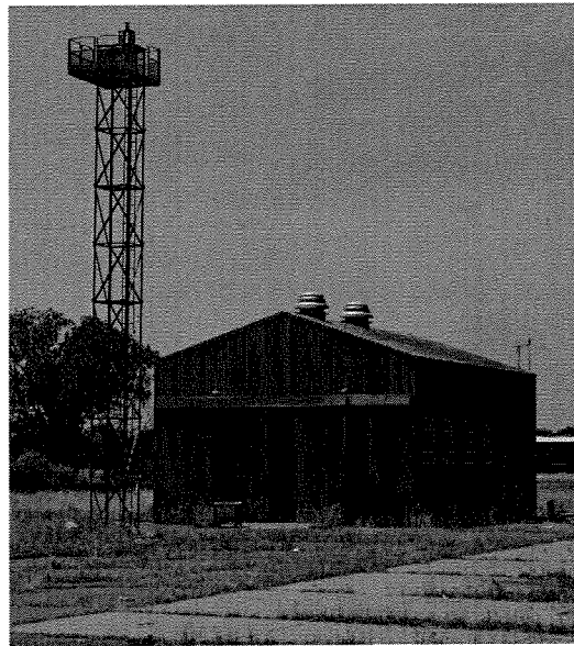
Plate 142: Shop for Test Stand No. 1 (Unit 124), Beta Test Complex, 1963-1964. TV camera stand, foreground left. Looking southwest. View of May 2005.
