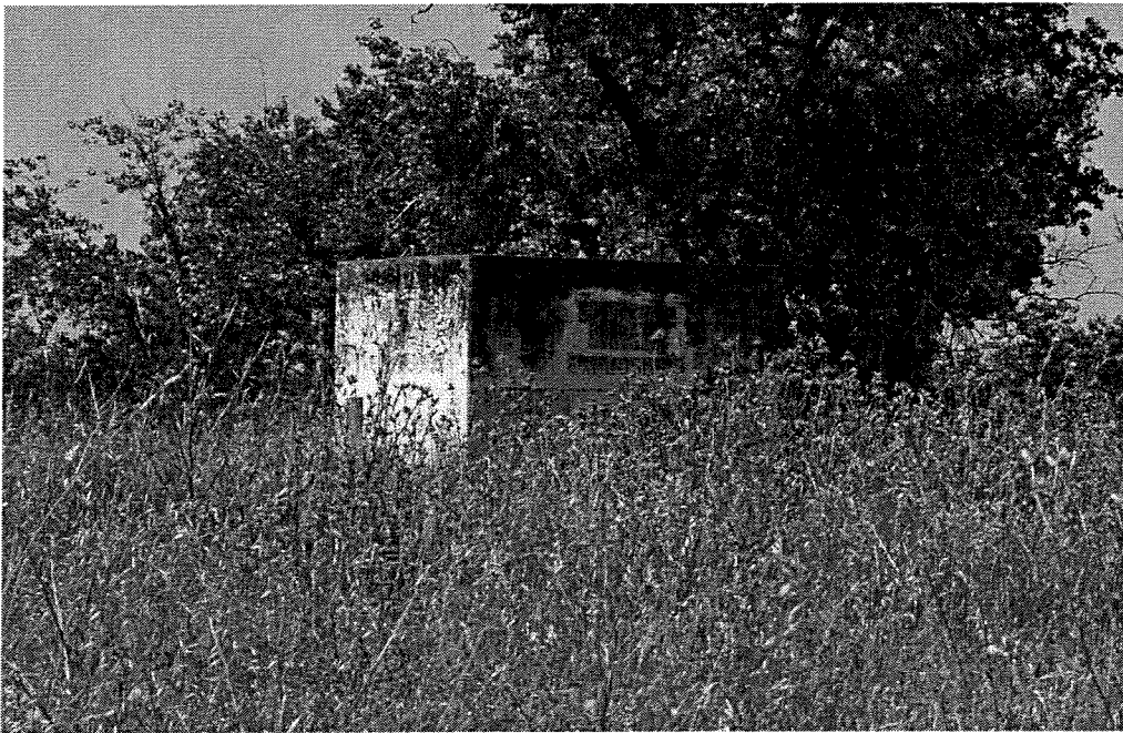
Plate 46: Personnel bunker, south/southeast of the original test site, Sigma Test Area, 1956. Looking southwest. View of May 2005.
