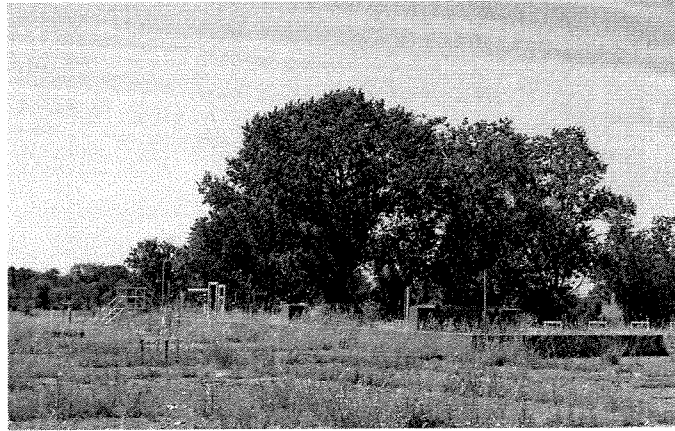
Plate 124: Liquid Hydrogen Tank at Test Stand No. 3 (Unit 147), Beta Test Complex, 1963-1964. Looking northwest. View of May 2005.
