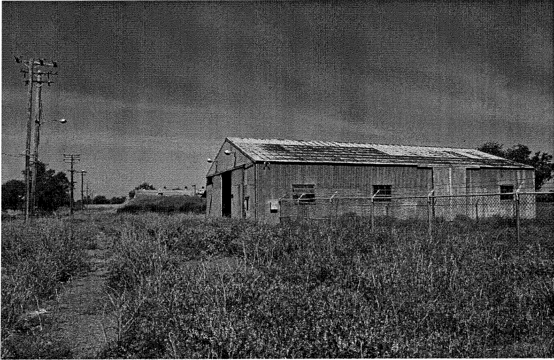
Plate 15: Storage Building (Unit 102), Assembly Building (Unit 103), and Motor Storage Building (Unit 104), Solid Propellant Assembly Area, 1956. East to west overview. Looking west. View of May 2005.
