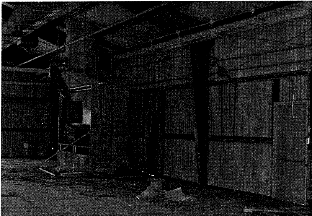
Plate 24: Assembly Building (Unit 103), Solid Propellant Assembly Area, 1956. Interior, looking northeast. View of May 2005.
