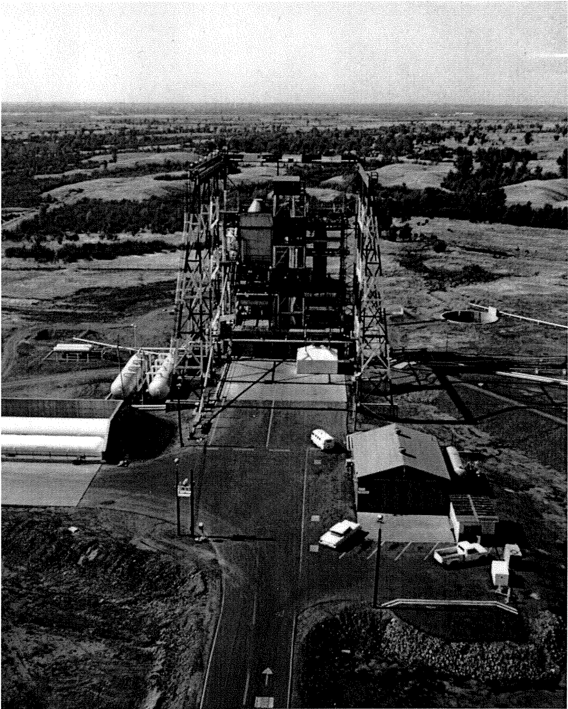
Plate 61: Test Stand No. 2, Alpha Test Complex, 1956-1957. Left to right in photograph: LOX tanks with barricade wall, steam accumulator tanks, test stand, shop (foreground), and deflector-water containment tank (background). Looking northwest. View of ca.1965. Courtesy of NASA.
