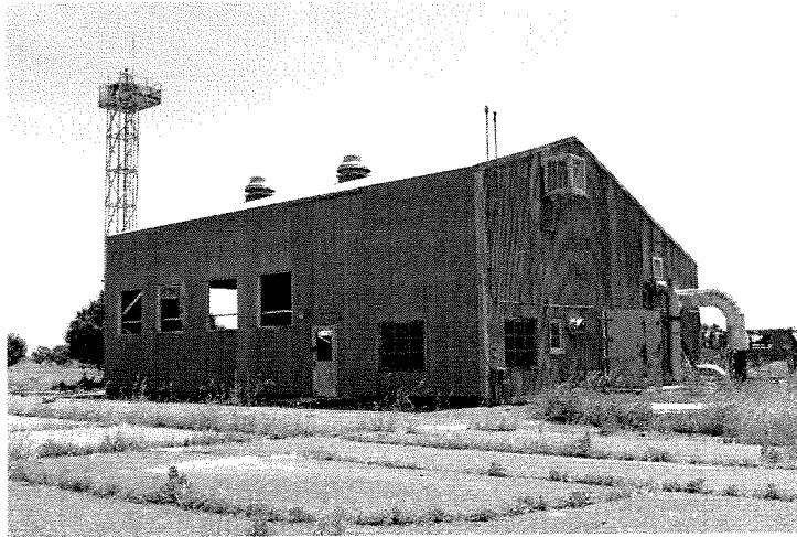
Plate 112: Shop for Test Stand No. 3 (Unit 133), Beta Test Complex, 1963-1964. TV camera stand, background left. Looking southeast. View of May 2005.
