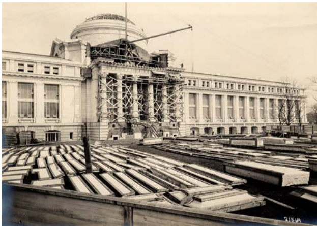
Construction of the U. S. National Museum, 1909.
