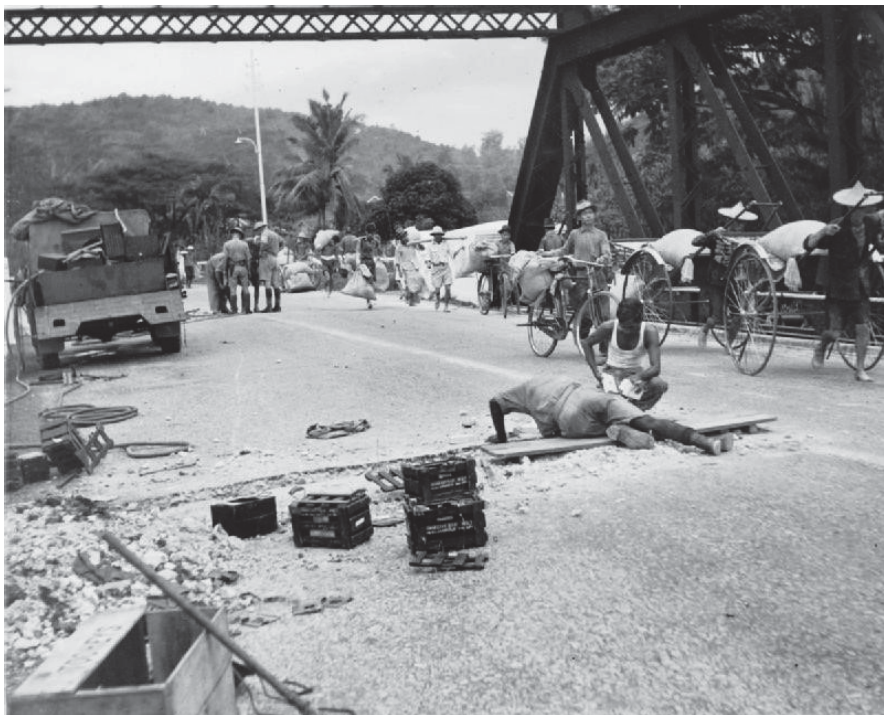
Figure 1. Royal Engineers preparing to blow up a bridge near Kuala Lumpur during retreat. From the collections of the Imperial War Museums, UK.
