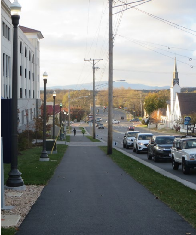
A completed Smart Scale project in Harrisburg, VA. Photo courtesy of Virginia's Office of Intermodal Planning and Investment.
