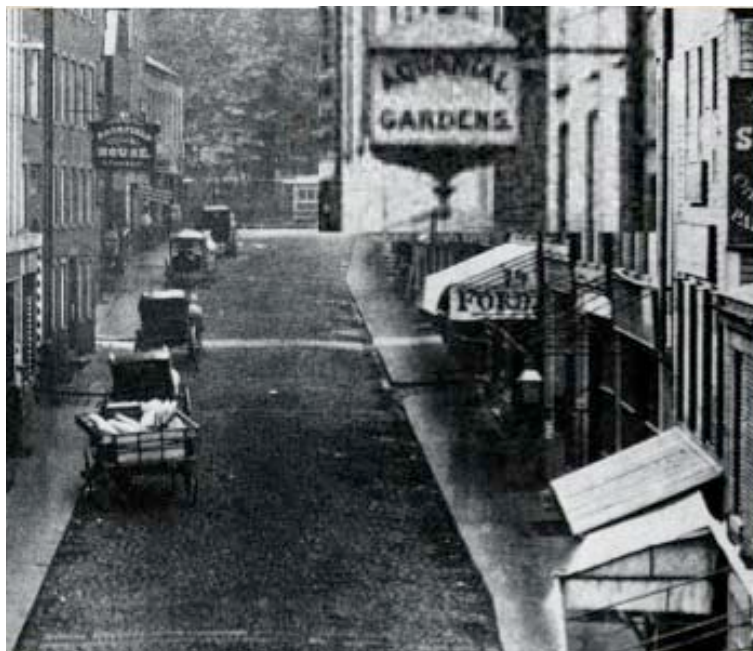
The Bromfield St. entrance of the Aquarial Gardens.
