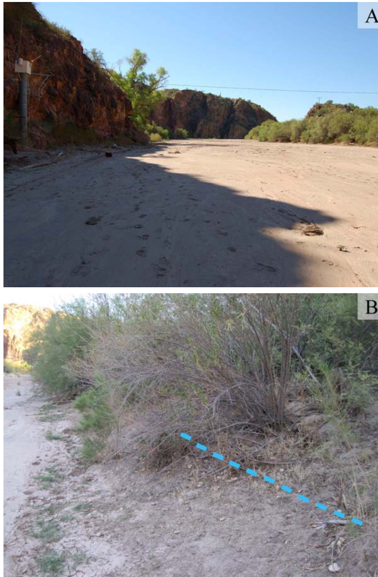
Figure 40. Hassayampa River, with the field OHWM shown by the blue dashed line: (A) channel confined by bedrock outcrops on the left bank and a railroad track on the right bank, and (B) vegetation below the railroad track, showing the slight increase in bank slope just below where shrubs are established along the channel bank.
