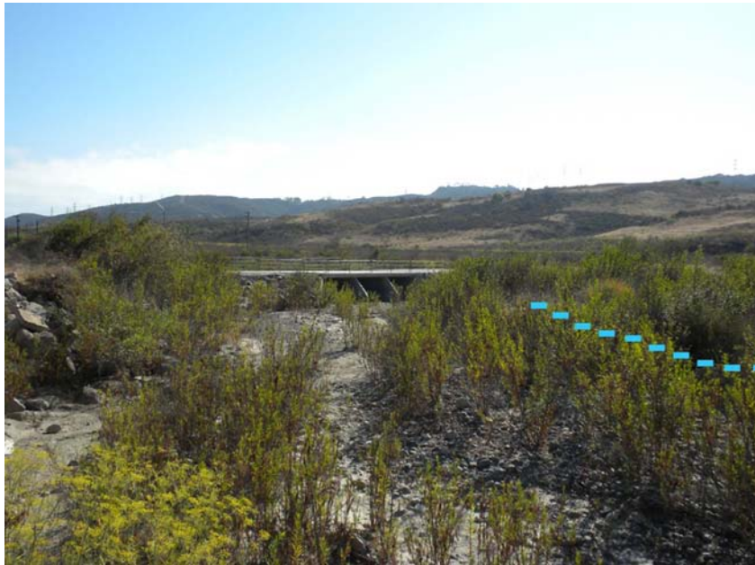
Figure 26. Cristianitos Creek, looking downstream towards the gage at the bridge. Flow extends outward from both corners of the bridge at an angle, and in higher flows the bridge may act as a dam-like confining structure. The OHW shown by the blue dashed line occurs at a break in slope that is associated with more dense vegetation and cobbles that are larger than the sediments in the active channel.
