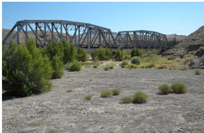
Figure 29. Gage at Mojave River, located beneath the railroad tracks. The channel flows between the riprap-supported railroad track banks and the mountainside.
