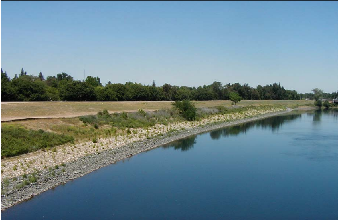
Figure 21. Site 4R on the American River after Bank Protection in 2001.
