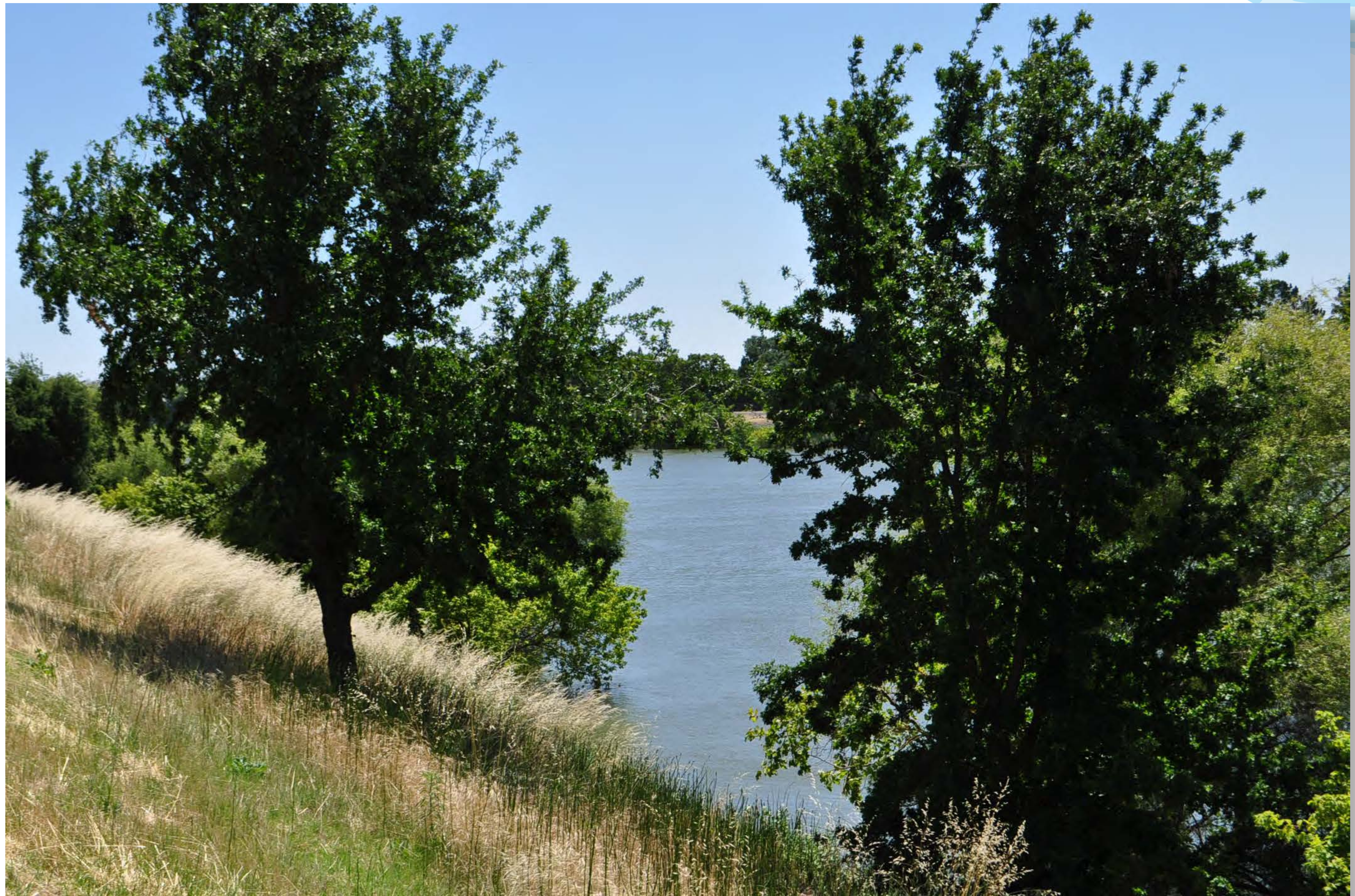
On South River Road, looking east and across the river toward Sacramento's Little Pocket neighborhood. This levee stretch is included in the 6 miles proposed for upgrades under the Southport Sacramento River EIP.
