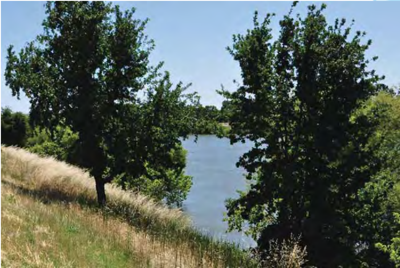
On South River Road, looking east and across the river toward Sacramento's Little Pocket neighborhood. This levee stretch is included in the 6.4 miles proposed for upgrades under the Southport Sacramento River EIP.
